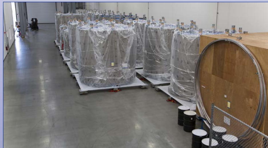
Conductor spools stored prior to winding
