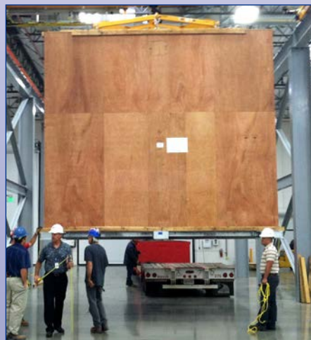
Unloading a conductor spool from the delivery
