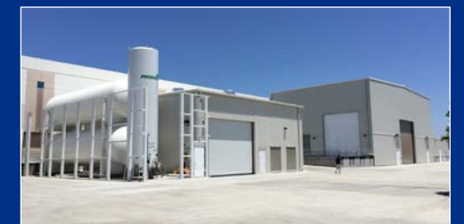
Final Test Facility
