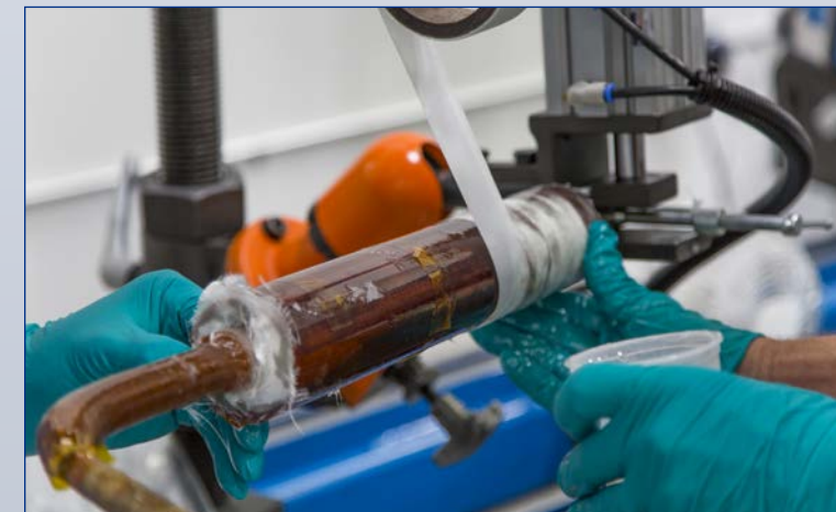
Thirty-nine helium pipes welded and insulated to provide the supply and return for supercritical helium at 4.7 K
