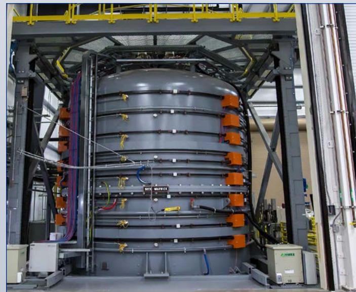
Furnace closed for module heat treatment
