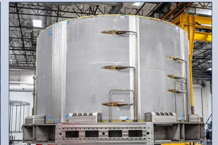
Module after piping installed
