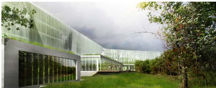
The architect's impression of the future ITER Headquarters building. This and other photos can be found in high-resolution on www.iter.org .
