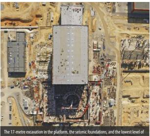
The 17-metre excavation in the platform, the seismic roundations, and the lowest level of the Tokamak Complex are no longer visible as contractors move forward on the Tritium, Tokamak and Diagnostics buildings.
