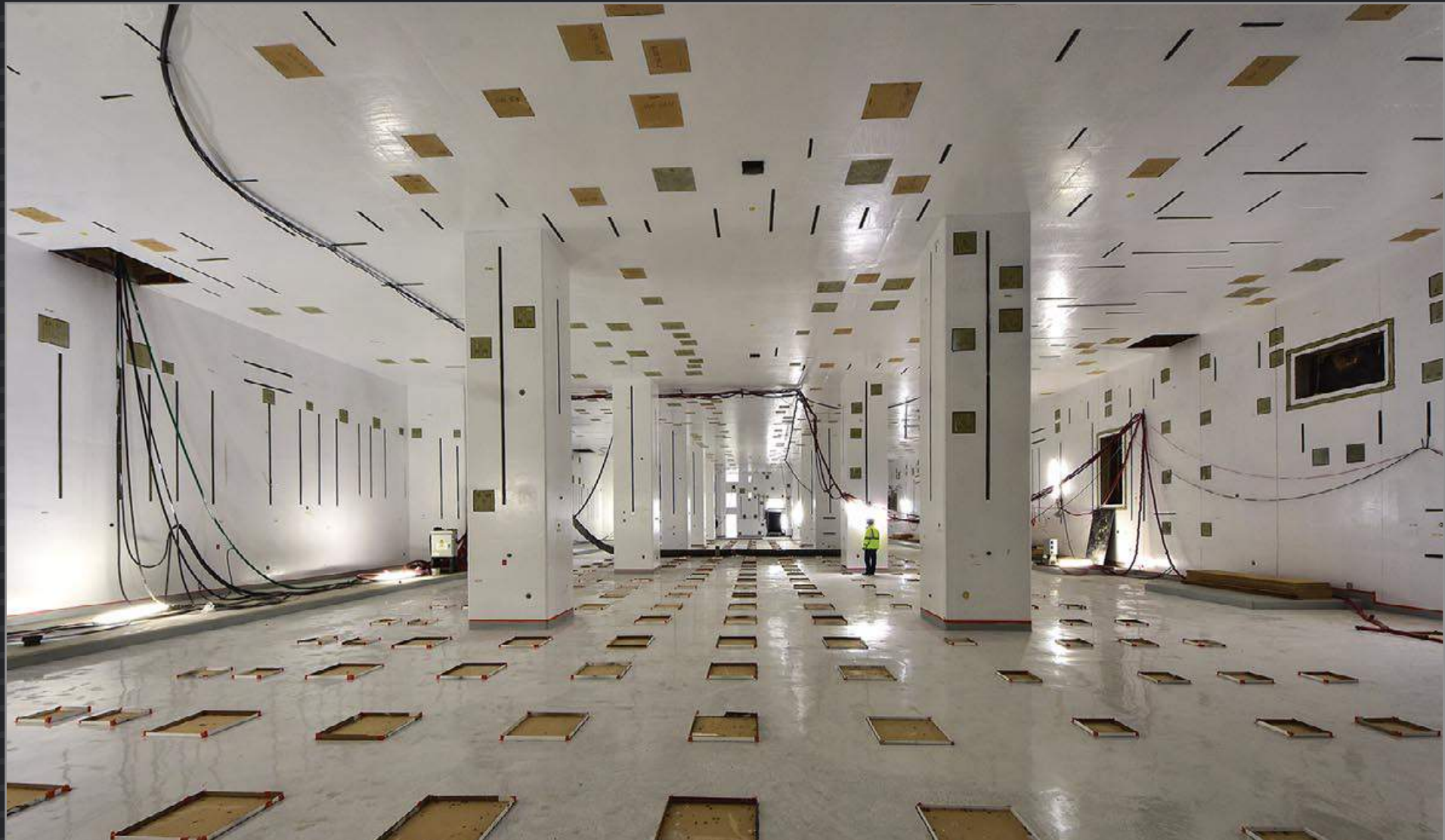
Now painted in white, the lowest basement level of the Diagnostic Building is ready for handover to contractors for systems installation. Embedded plates – for the attachment of system supports – are visible on all surfaces. December 2018
