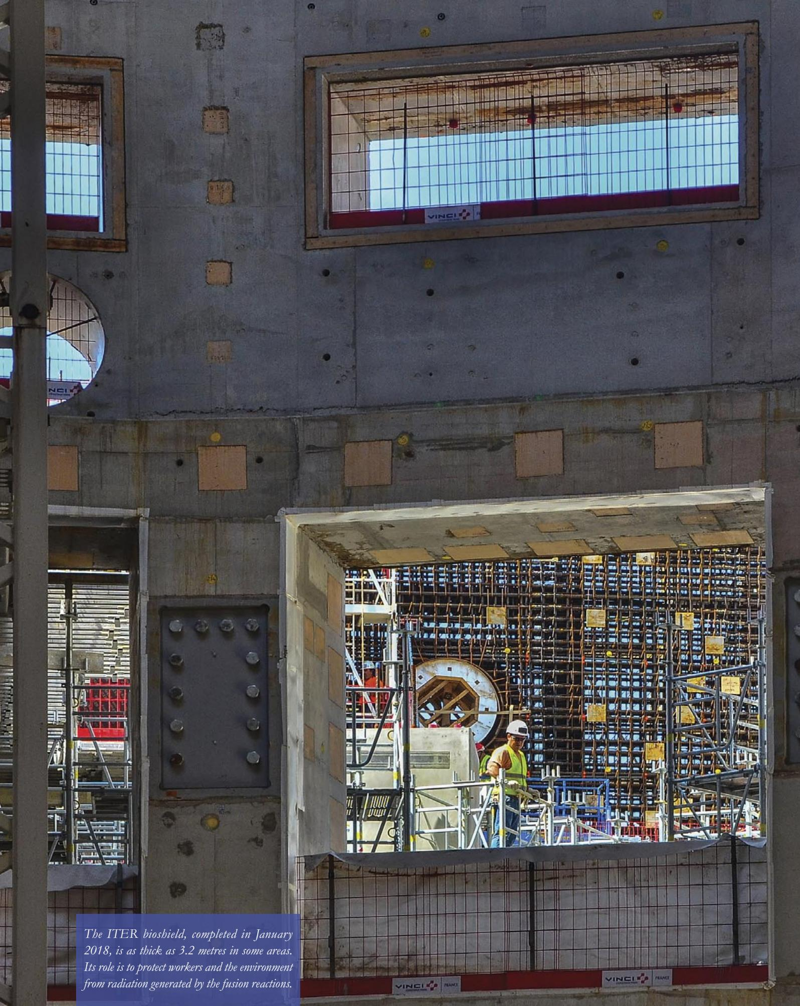
*The ITER bioshield, completed in January 2018, is as thick as 3.2 metres in some areas. Its role is to protect workers and the environment from radiation generated by the fusion reactions.*
