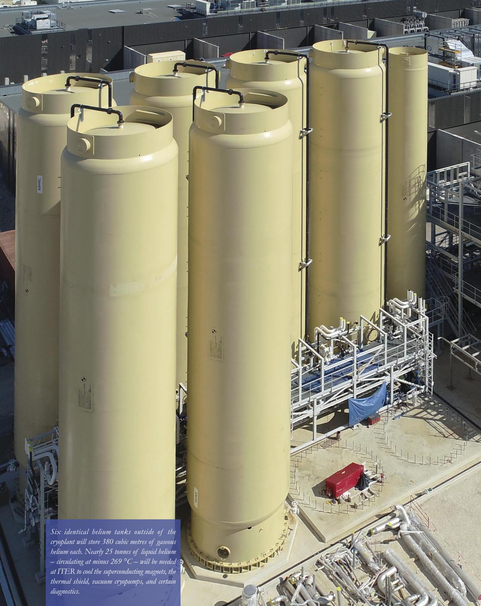
*Six identical helium tanks outside of the cryoplat will store 380 cubic metres of gaseous helium each. Nearly 25 tonnes of liquid helium – circulating at minus 269 °C – will be needed at ITER to cool the superconducting magnets, the thermal shield, vacuum cryopumps, and certain diagnostics.*
