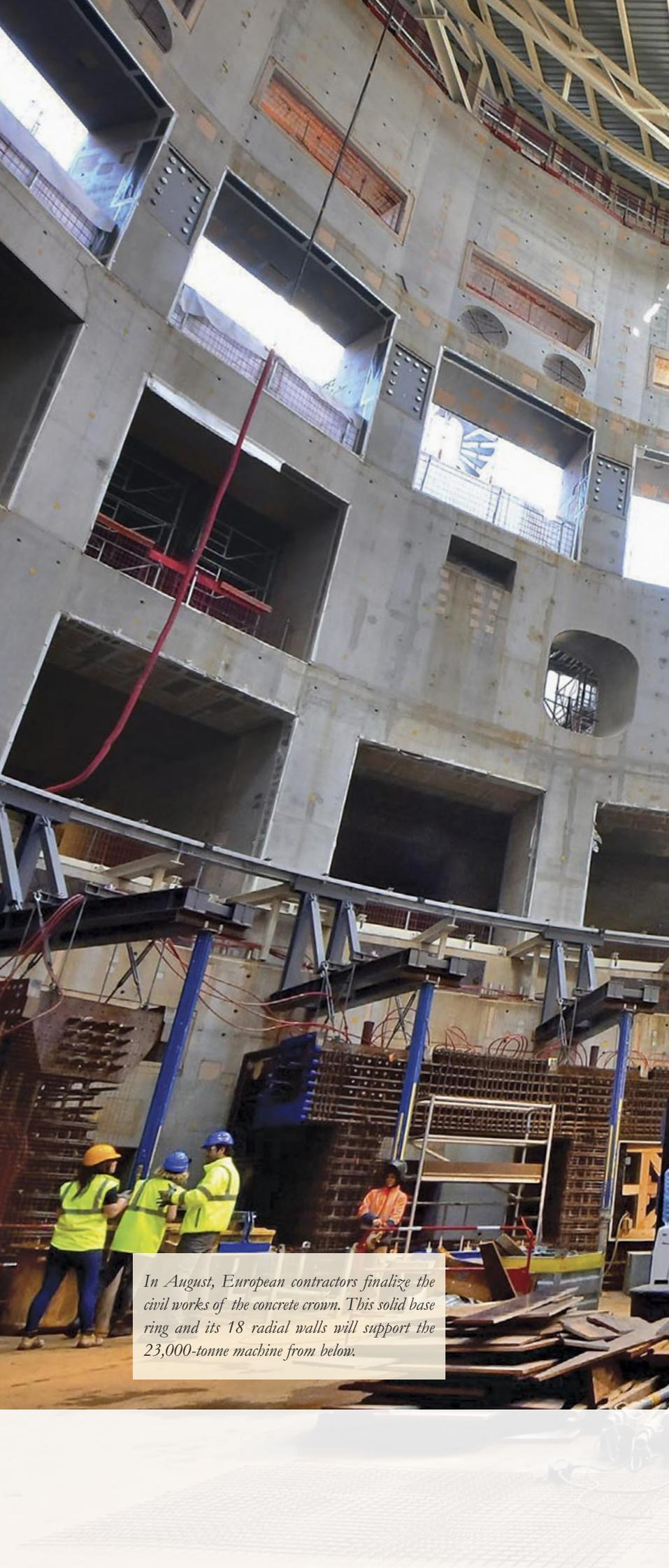
*In August, European contractors finalize the civil works of the concrete crown. This solid base ring and its 18 radial walls will support the 23,000-tonne machine from below.*
