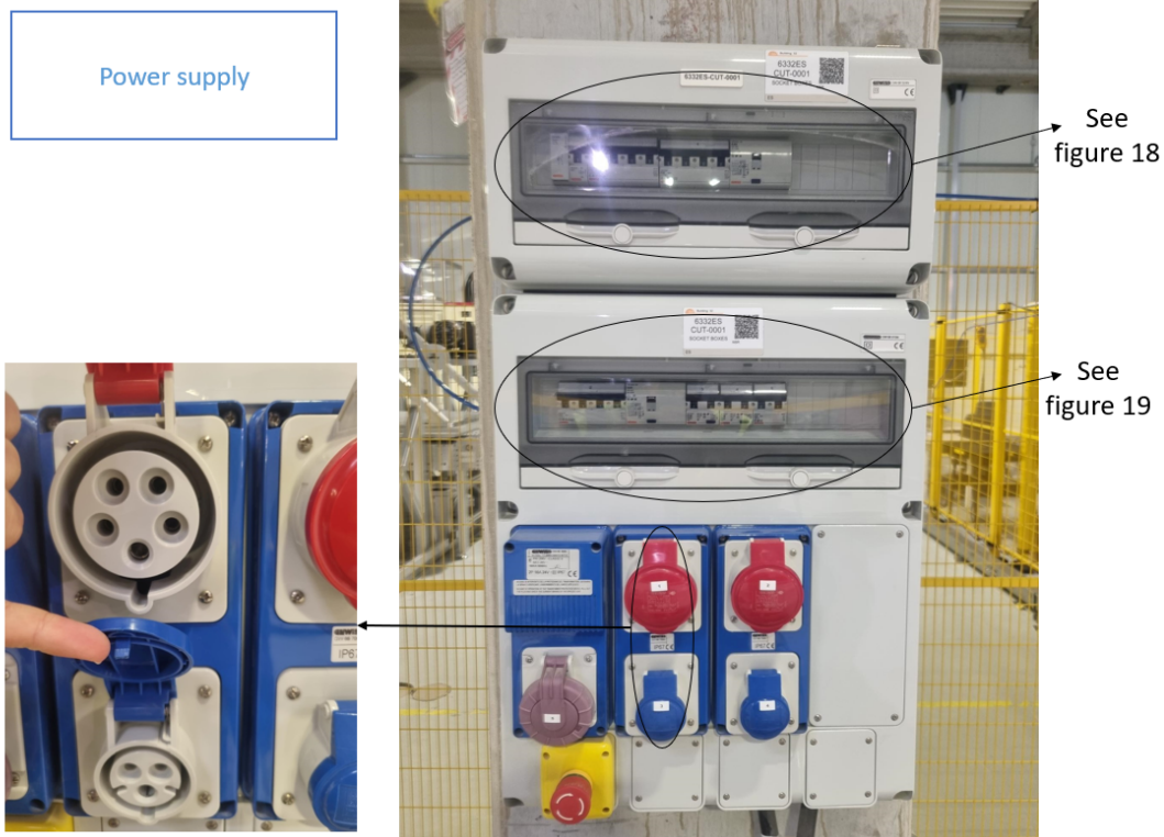
Figure 17 Power supply 32 A – 16 A
