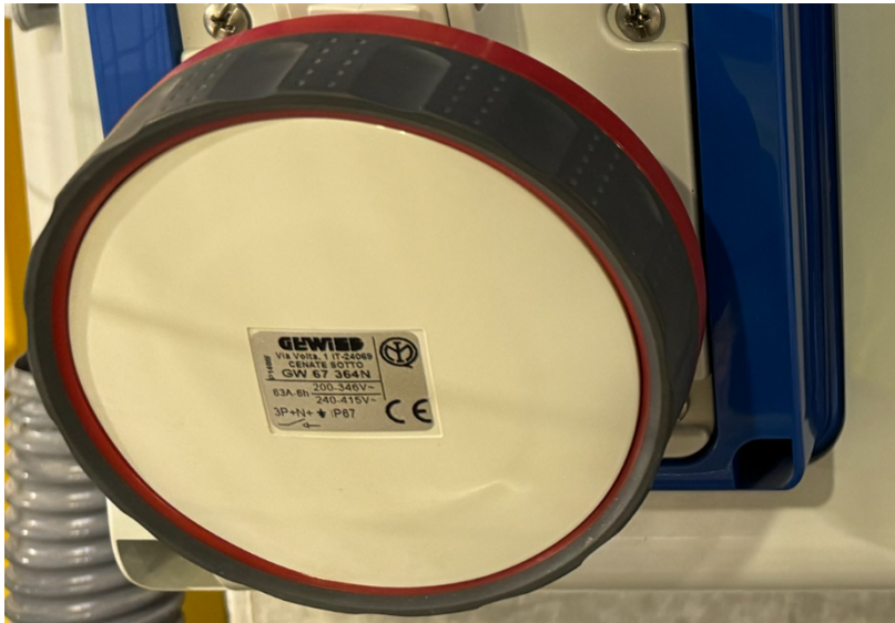
Figure 21 Socket power supply 63 A
