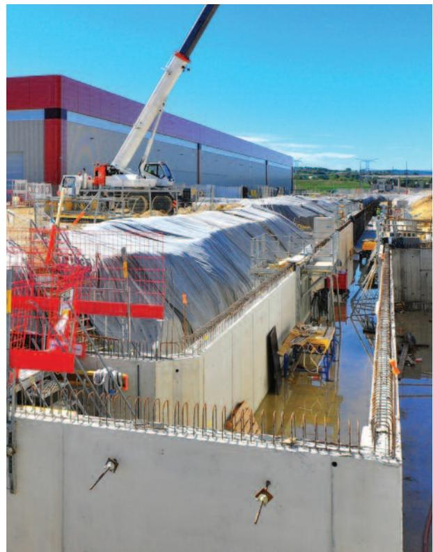
*Underground galleries like this one crisscross the platform to deliver industrial services to all the buildings of the ITER plant.*
