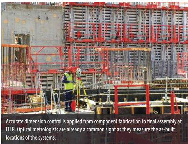
Accurate dimension control is applied from component fabrication to final assembly at ITER. Optical metrologists are already a common sight as they measure the as-built locations of the systems.
