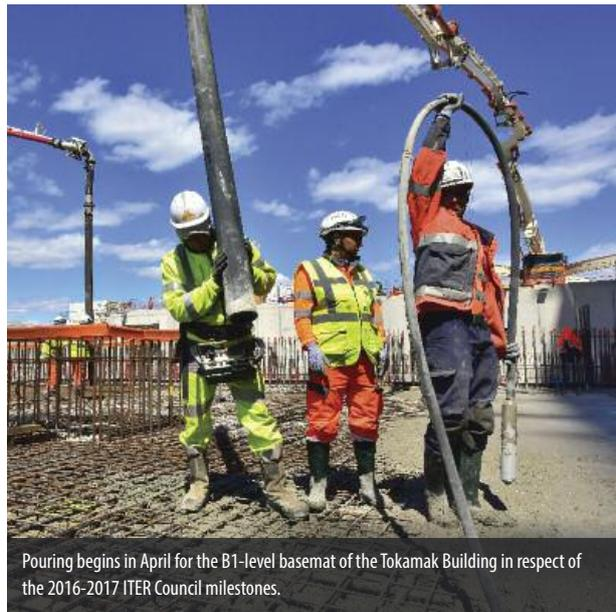
Pouring begins in April for the B1-level basemat of the Tokamak Building in respect of the 2016-2017 ITER Council milestones.
