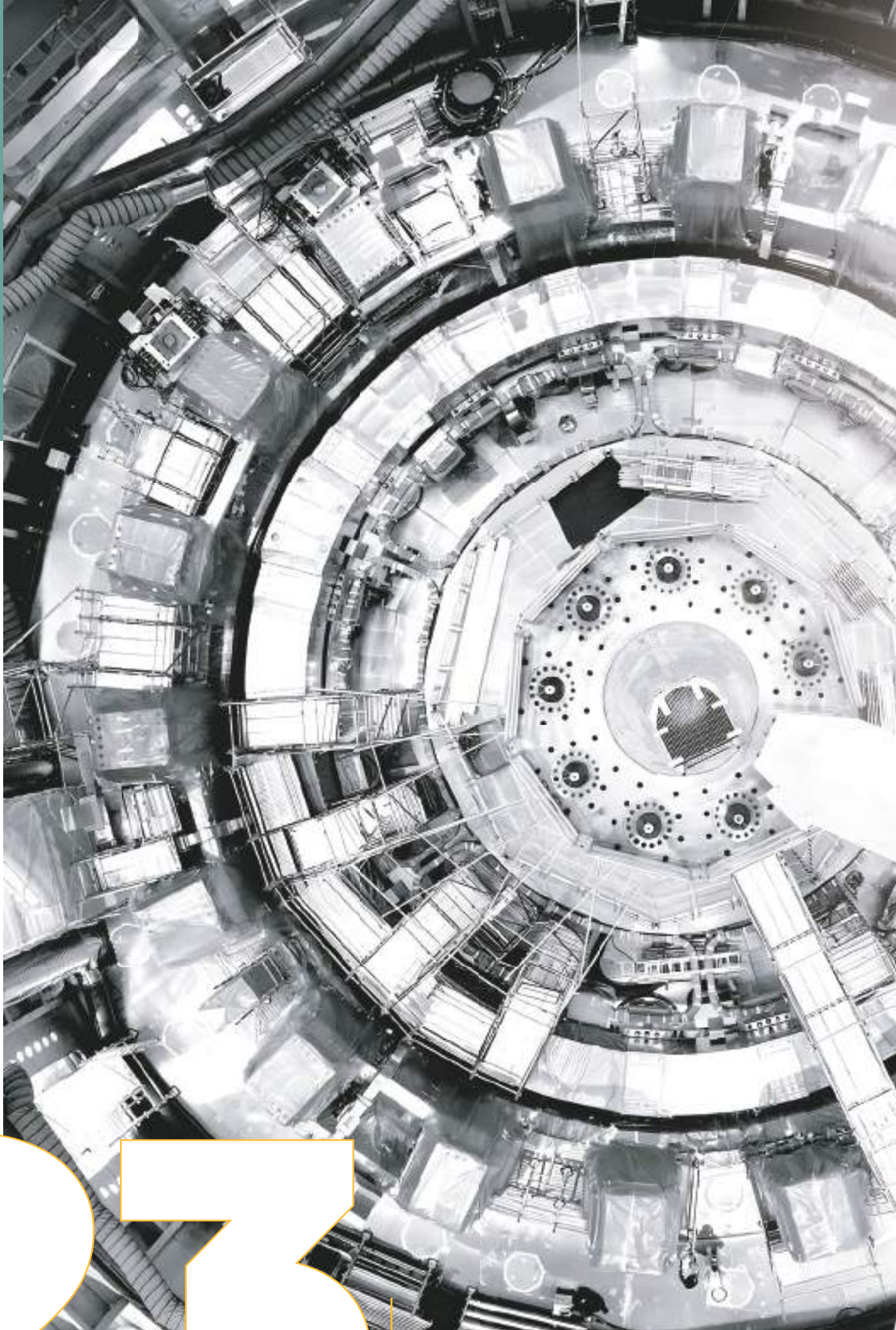
The nine sector modules of the ITER vacuum vessel will be lowered into this cylindrical space, clamped, and welded. The ITER Organization is considering nine-sector simultaneous welding as a way to reduce weld deformation.
