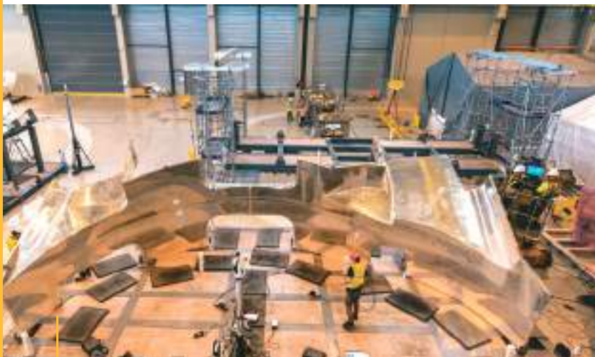
An outboard segment of thermal shield is surveyed before transfer to contractors for repair or refurbishment.
