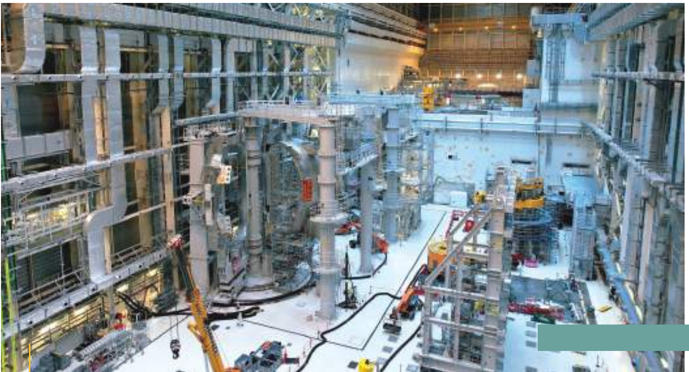
Looking towards the wall that separates the Tokamak pit from the Assembly Hall. In addition to the vacuum vessel sectors in tooling, two modules of the central solenoid can be seen stacked at right.
