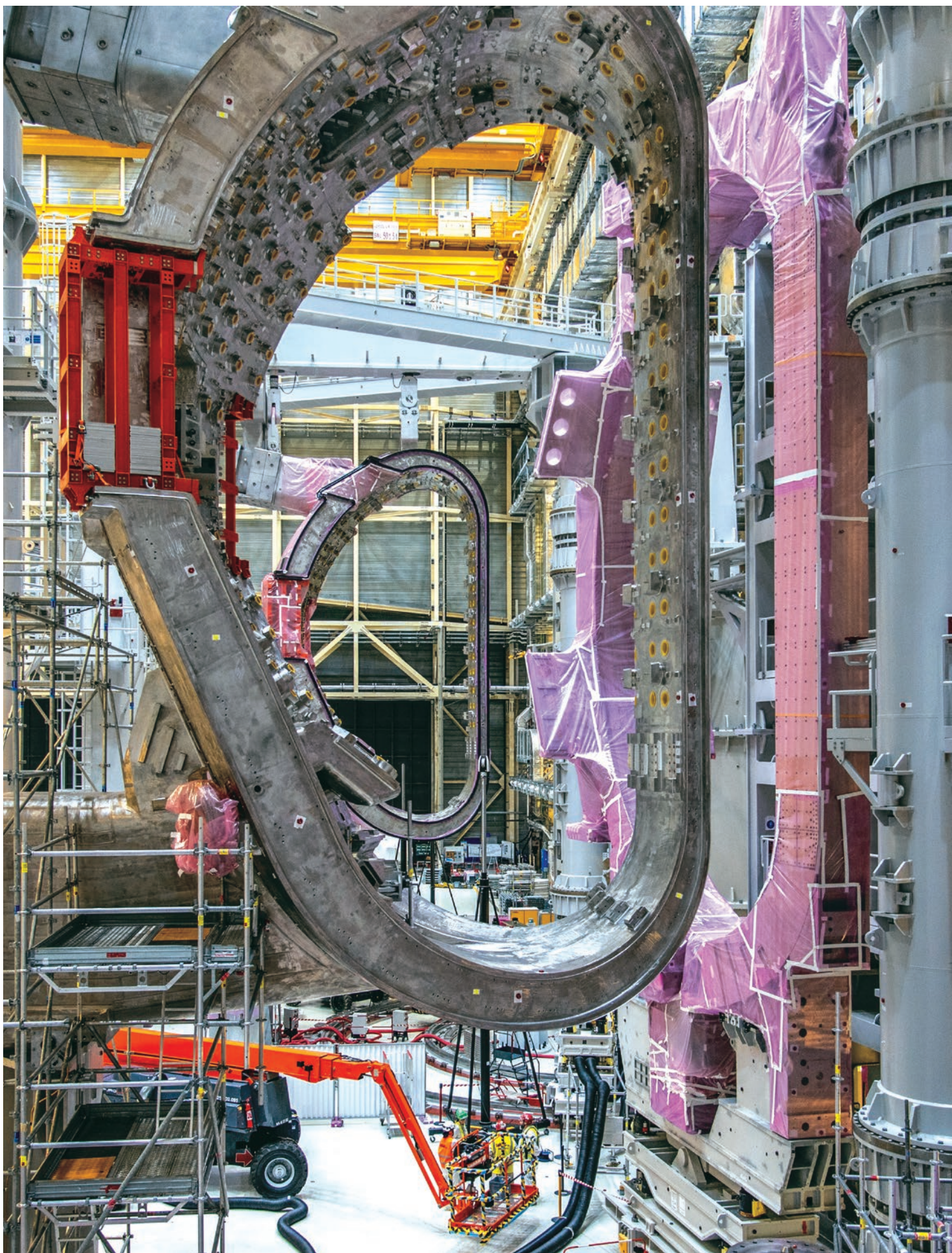
▲ Before repair work begins on sectors #7 and #6, the modules have to be disassembled. Here, toroidal field coils have been removed to the wings of the large tools and protected in pink plastic (February).
