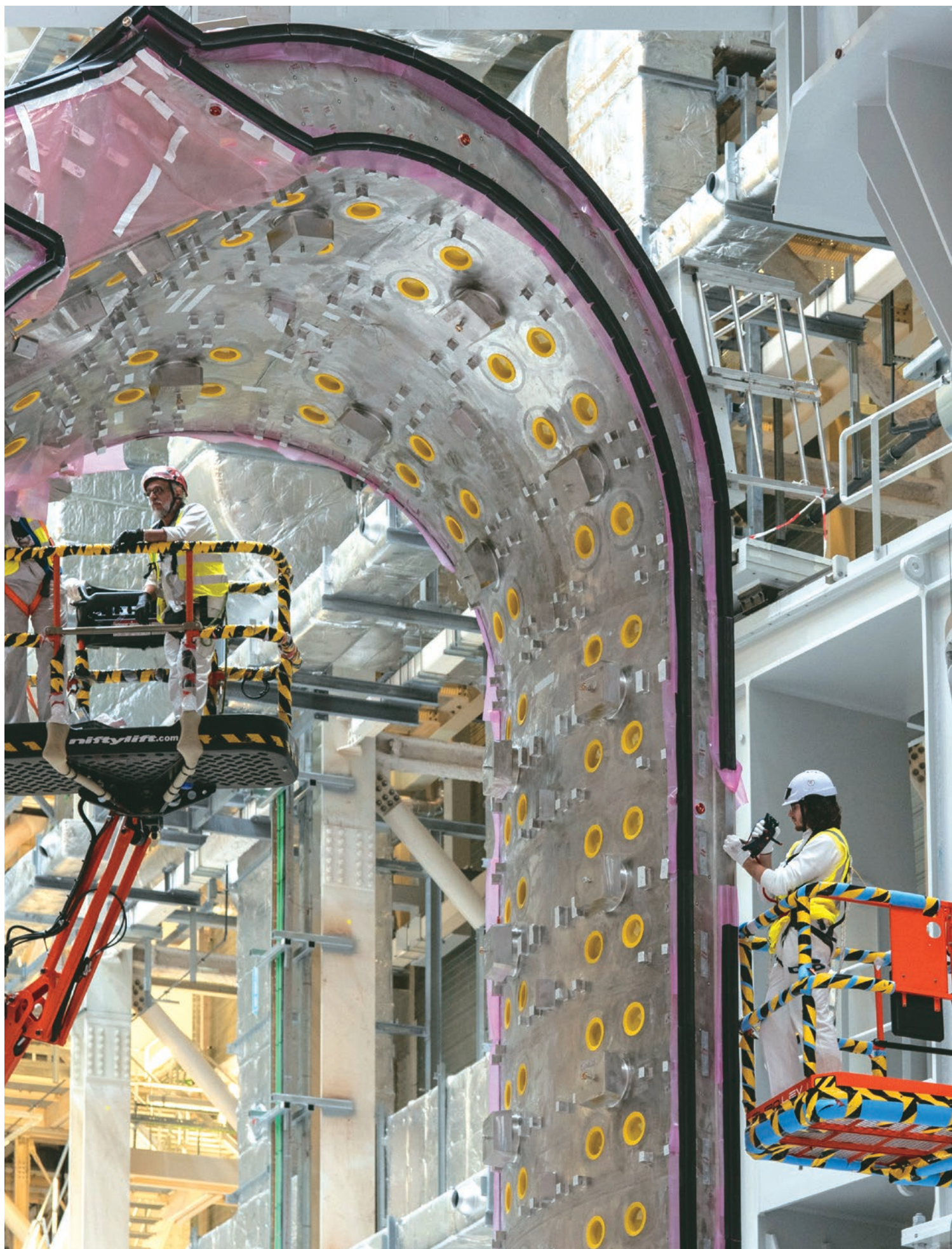
▲ In order to precisely identify the bevel regions that need to be rectified (outlined in black), metrologists perform ultra-precise measurements on both sides of vacuum vessel sector #7.
