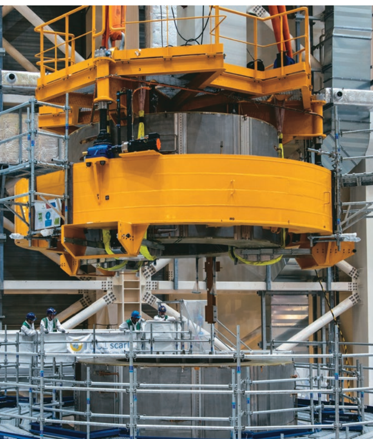
▲ A cylindrical magnet is added to the central solenoid stack in the Assembly Hall.
