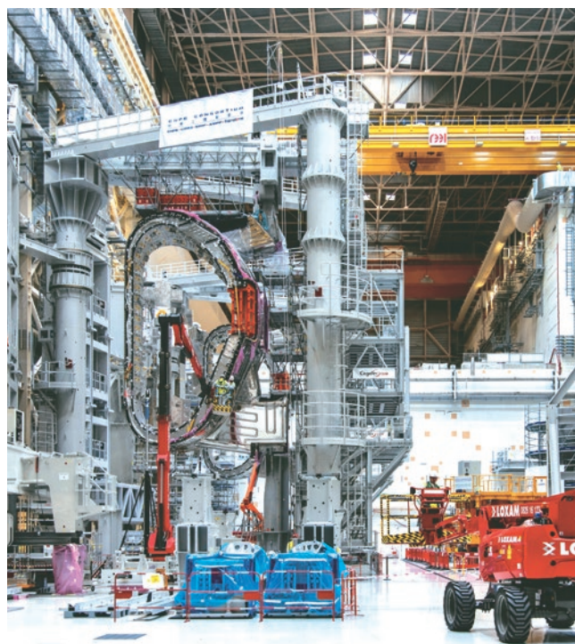
▲ Vacuum vessel assembly restarts in September, after repairs are completed on sector #7.
