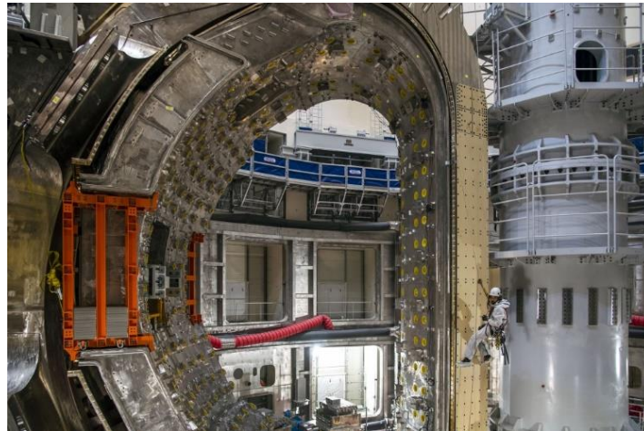
Fig.3. 5. The first sector of the ITER vacuum vessel was installed in May 2022. In-situ repairs were planned due to deviations from the allowable tolerance of the field joints but its qualification for the repair welding was not possible. Subsequently, the sector had to be removed from the pit in July 2023 for repair in 2024 [5].
