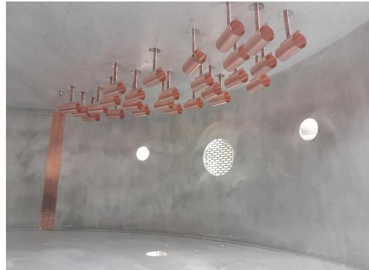
Internal view cavity showing coupling loops and transmission line
