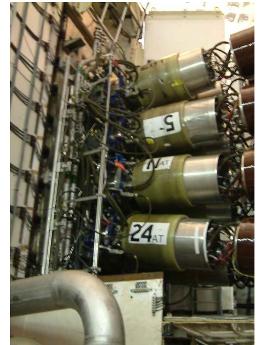
Neutraliser integrated with each ion source at JET
