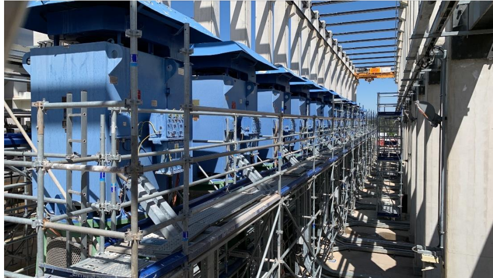
Vertical Pumps for HRS in Operation
