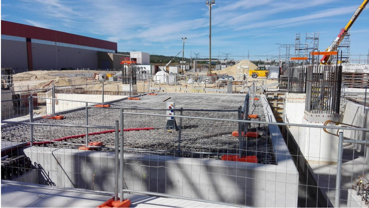
Cryoplat during civil works execution
