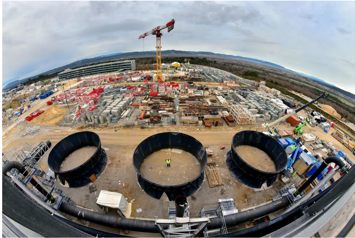
Heat rejection system during assembly
