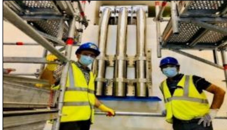
NFM7# support Frame installed at ITER in 2020
