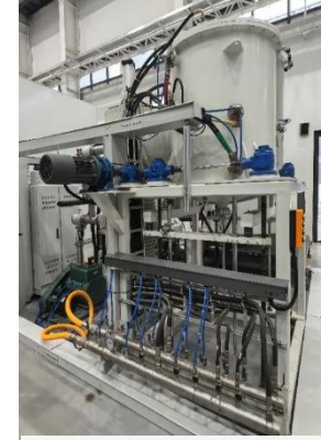
Welding Process Platform
