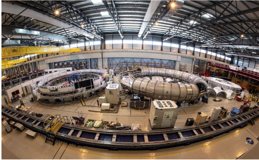
Fig. 6.1-57: PF Coil Manufacturing Underway at ITER Site, PF5 (far left), PF2 (left middle), test cryostat (empty, right middle), PF6 (far right).
