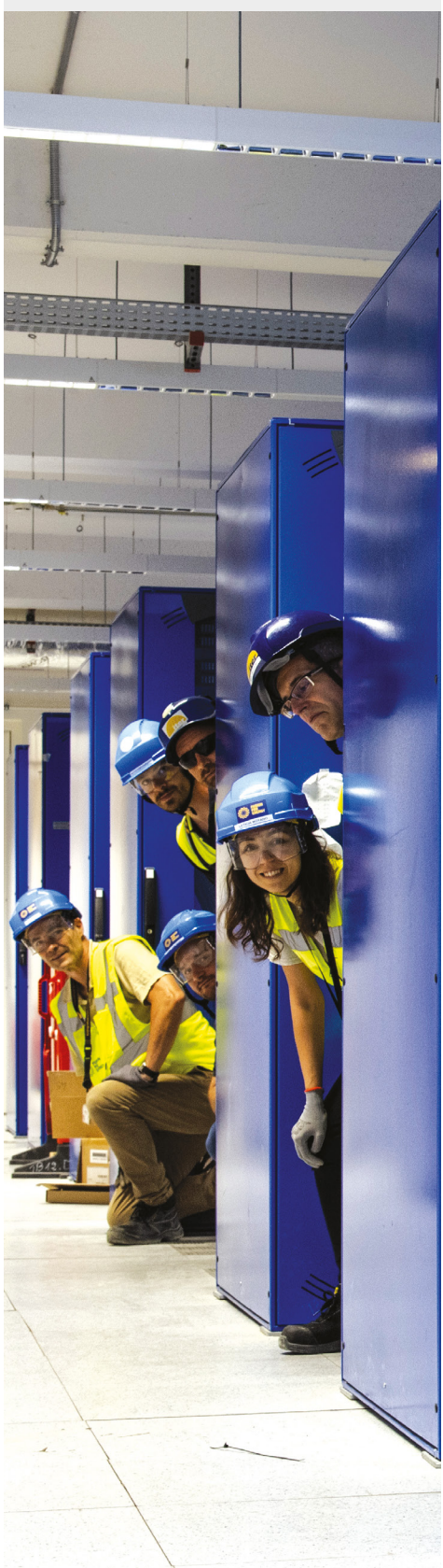
▲ Installing the cubicles that will orchestrate approximately 5 million "variables" during machine operation.
