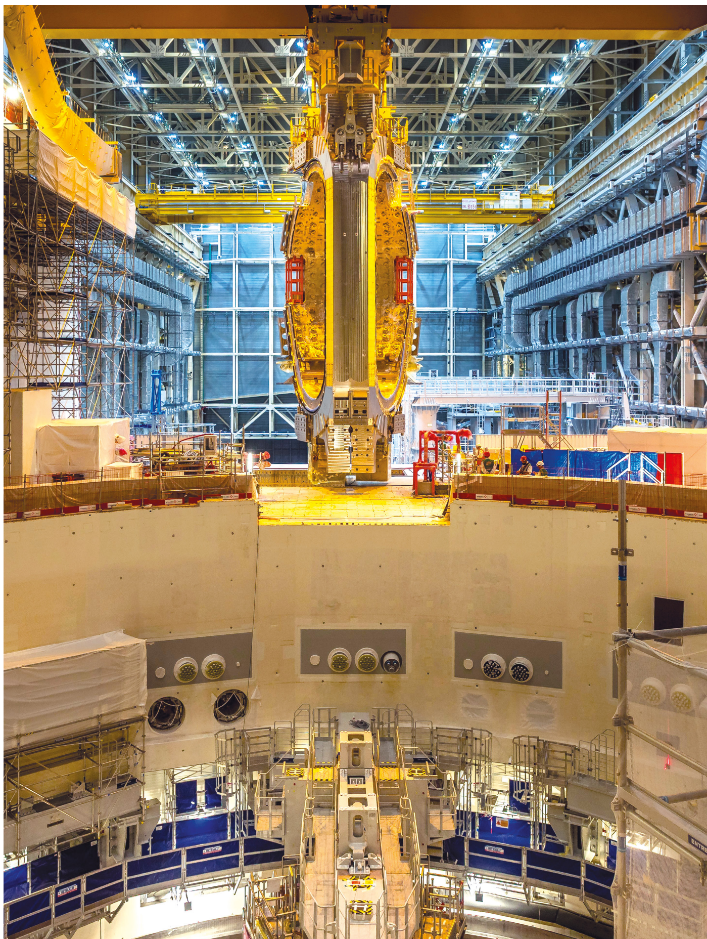
▲ A second vacuum vessel sector module is installed in the tokamak assembly pit in June.
