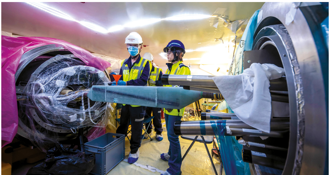
▲ Deep in the galleries of the Tokamak Building, segments of magnet feeders—which transport power and cryogens to the ITER magnets—are being connected.
