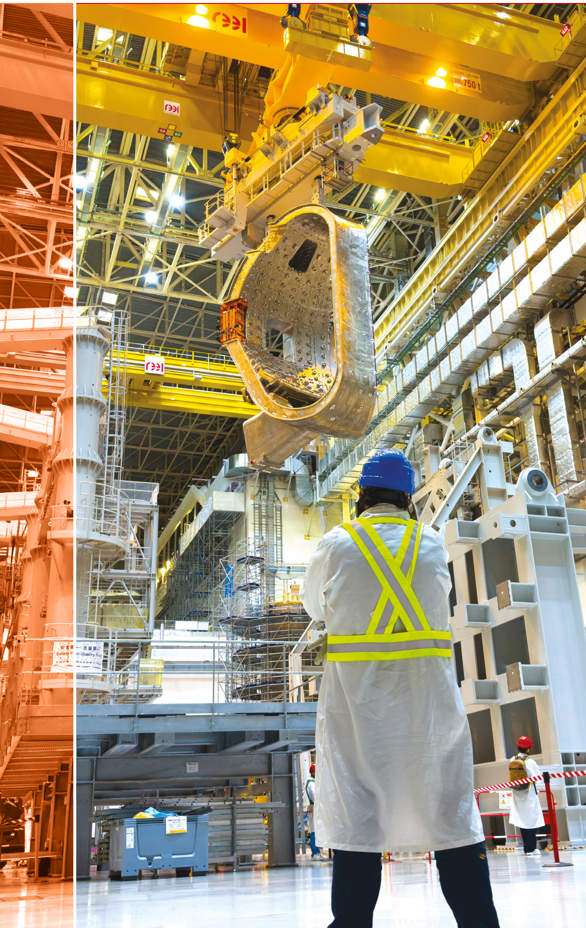
▲ Large tokamak components like this vacuum vessel sector are handled in the Assembly Hall by the powerful 1,500-tonne bridge cranes.
