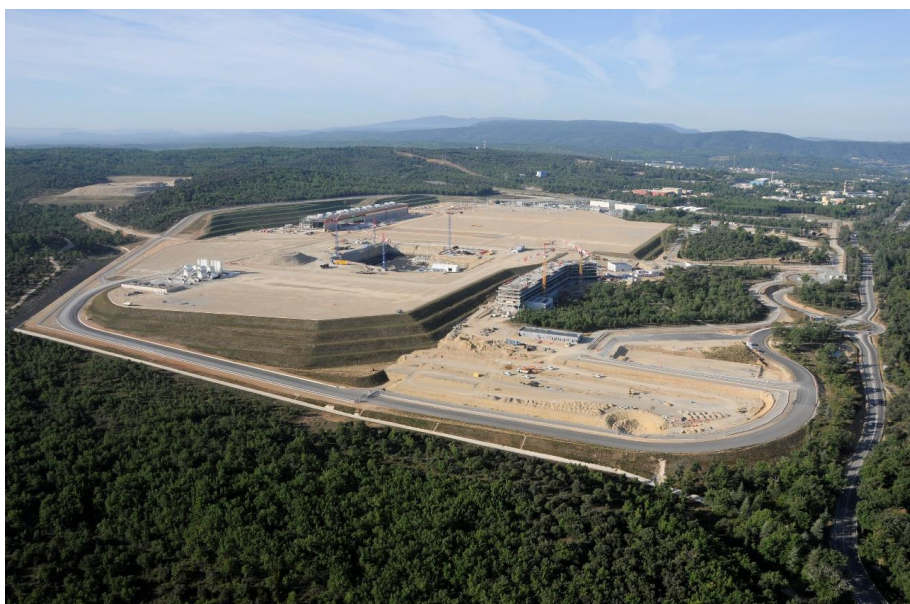
Fig. 8.4-18: Aerial Photo of ITER site, September 2011.
