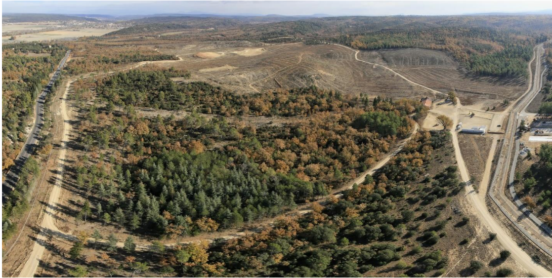
Fig. 8.4-1: ITER construction site, Cadarache- view toward Vinon-sur-Verdon.
