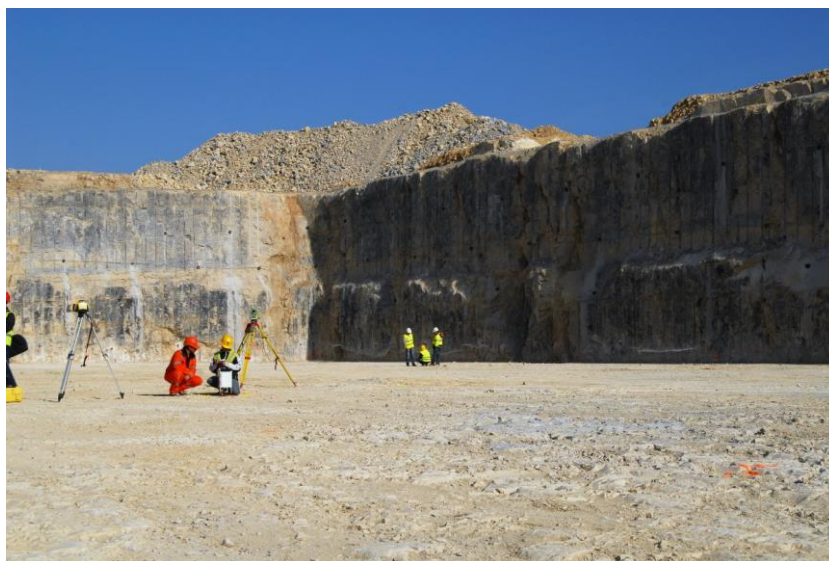
Fig. 8.4-12: The Tokamak Seismic Isolation Pit, seventeen metres below the surface of the ITER platform, May 2011.
