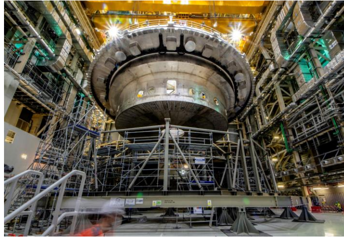
Fig. 8.4-42: Between the overhead heavy lift cranes and the component are yellow "spreader beams" that share the weight of the component and eliminate any tilt.
