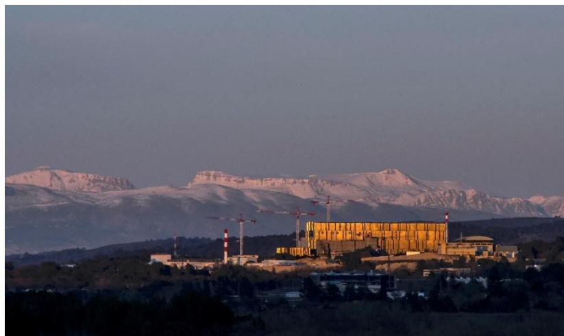
Fig. 8.4-48 : Aerial view of ITER site, late afternoon.
