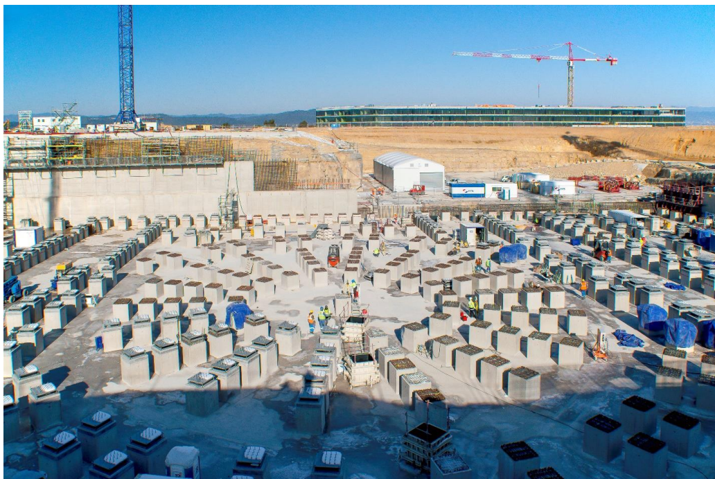
Fig. 8.4-16: Work on the seismic pads progresses, February 2012.
