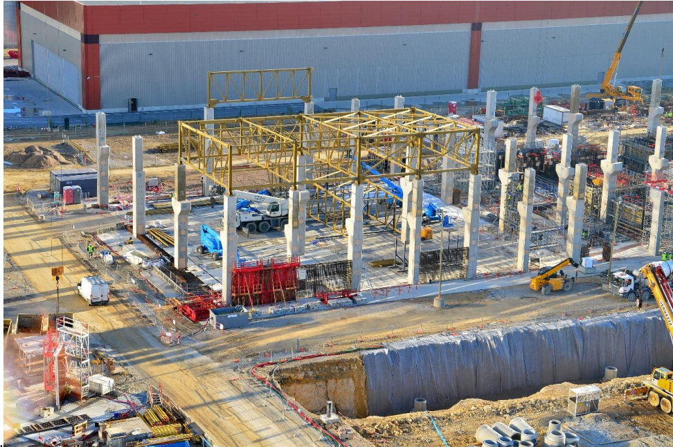
Fig. 8.4-34: Cryoplat construction is progressing as the roof frame is being positioned.
