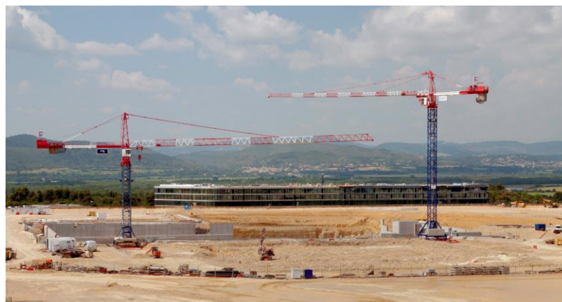
Fig. 8.4-20: Excavation Assembly Hall: Vast antechamber to the Tokamak Building.
