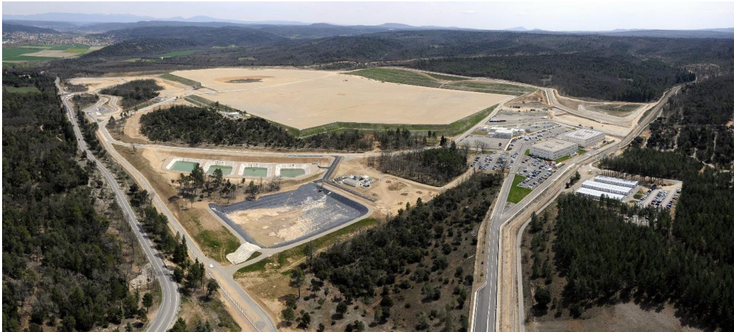
Fig. 8.4-3 : Panoramic photo, taken in September 2010, showing the ITER site as the digging begins for the Tokamak Complex.
