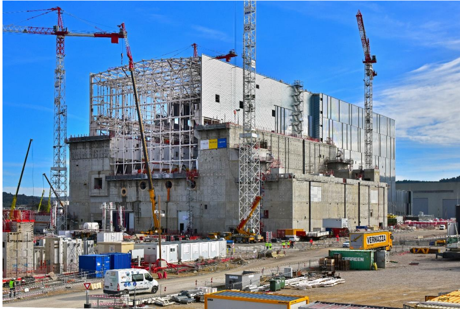
Fig. 8.4-27 : Frame of the crane hall nearly complete and a first layer of cladding now covers the south wall and part of the roof, January 2020.
