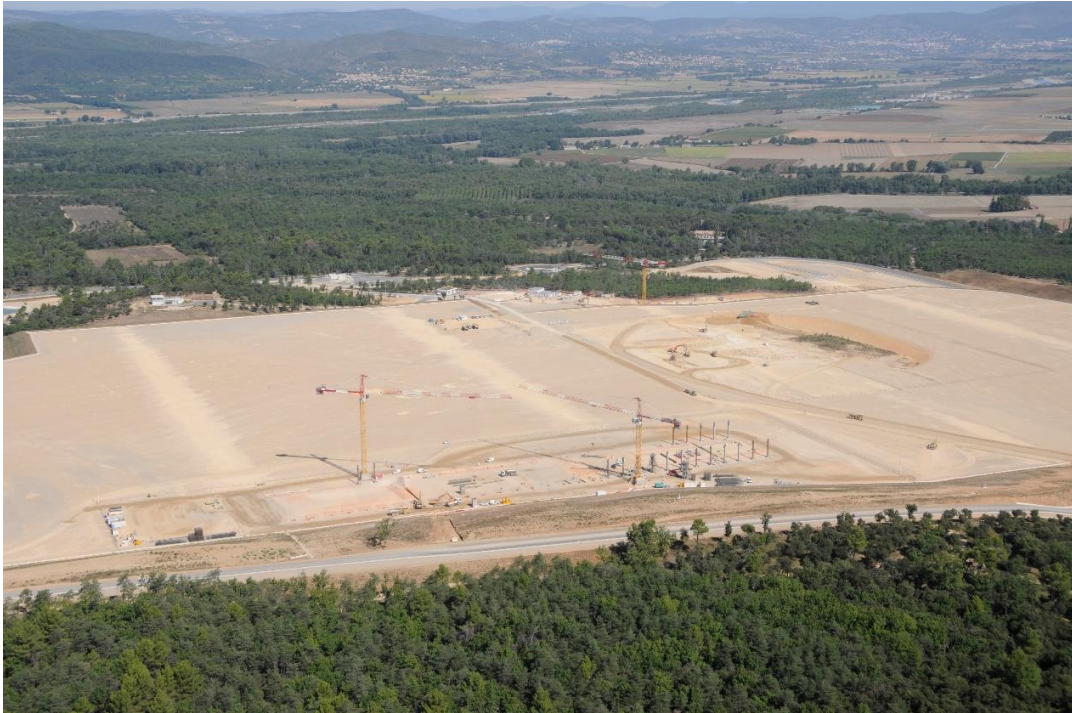
Fig. 8.4-7: The Poloidal Field Coil Winding Facility under construction, view from above.
