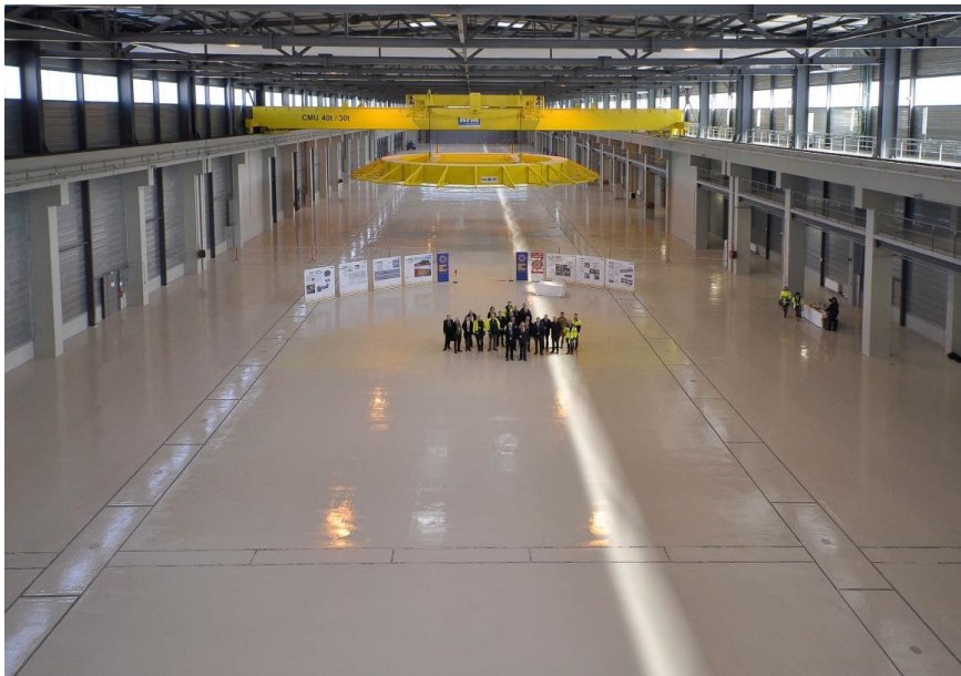
Fig. 8.4-10: PF Winding Facility completed.
