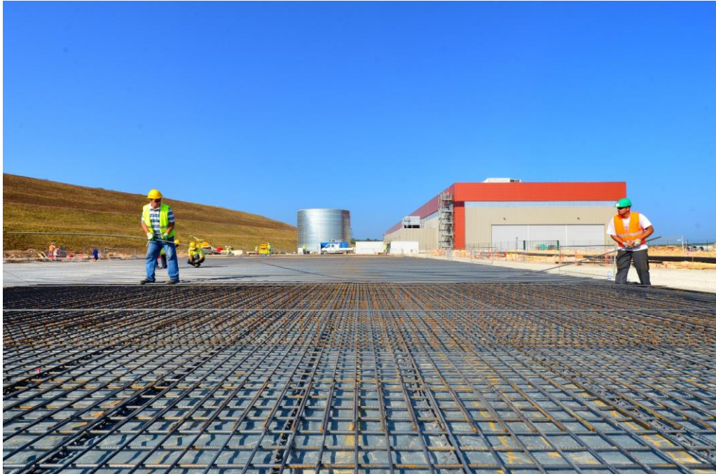
Fig. 8.4-40: Workers complete rebar operations on the 5,500 square-metre slab of the Cryostat Workshop, adjacent to the Poloidal Field Coils Winding Facility, July 2013.
