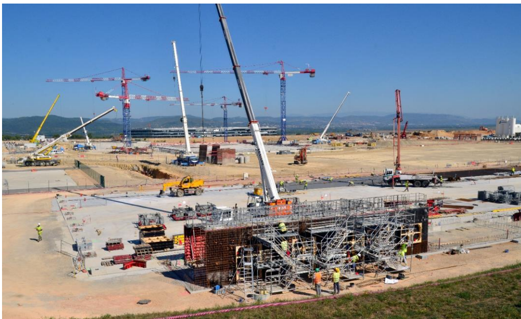
Fig. 8.4-39: Adjacent to the Cryostat Workshop, the ancillary building under construction will house offices, machinery, power supplies and other utilities, August 2013.
