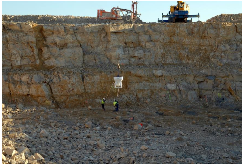
Fig. 8.4-11:: excavation of the Tokamak Seismic Isolation Pit, December 2010.
