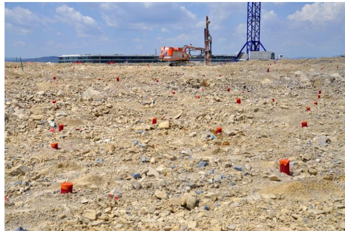
Fig. 8.4-19: Excavation work for the future Assembly Hall, 500 holes drilled down to 7 metres to profile the rock substrata.
