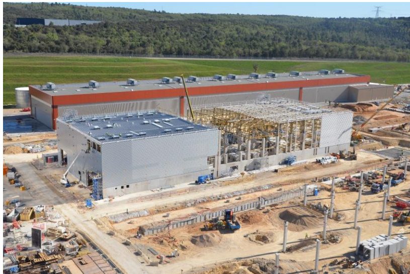
Fig. 8.4-37: Cryoplant building's cladding nearly finalized and work is underway to pour the ground slab for the exterior storage area.
