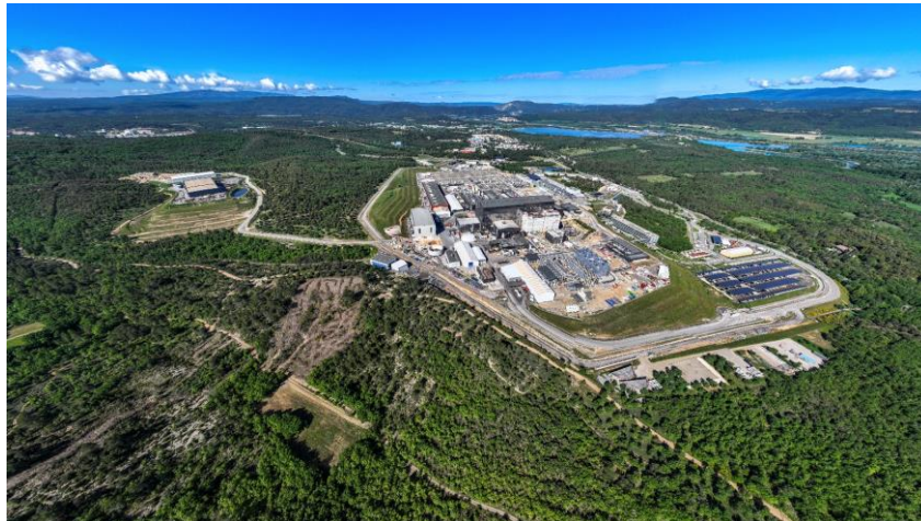
Fig. 8.4-47 : Aerial view of ITER site, May 2025.
