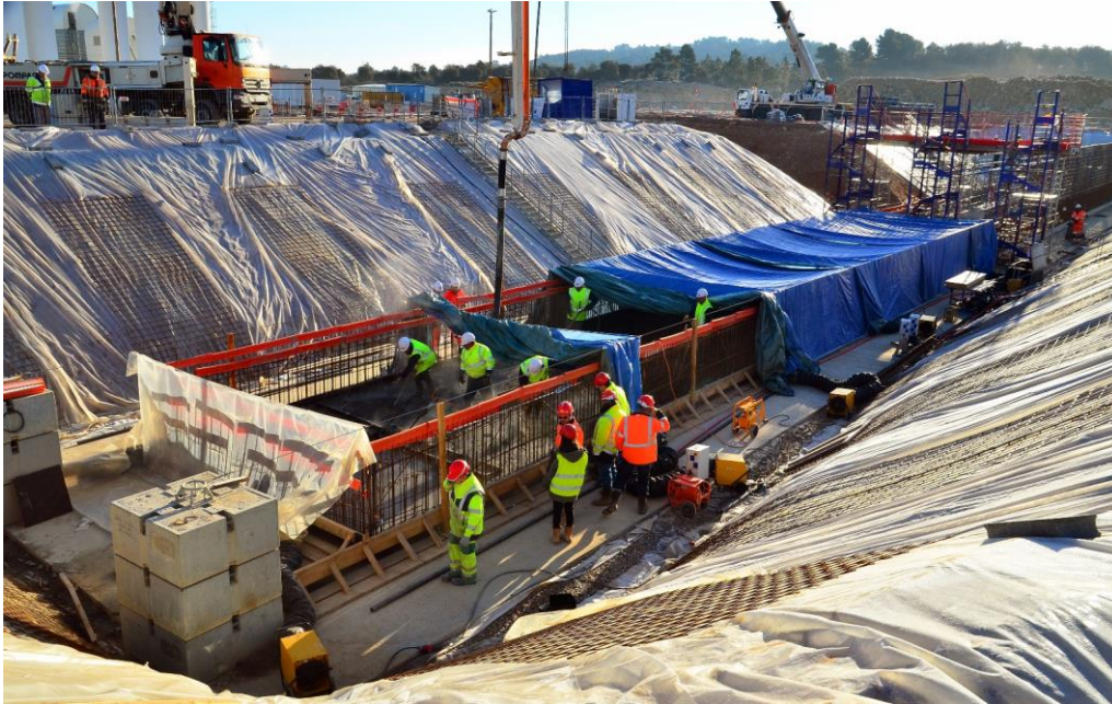
Fig. 8.4-28 :Site Services Building construction, it will accommodate and distribute a large number of industrial support services that are indispensable for operating ITER.
