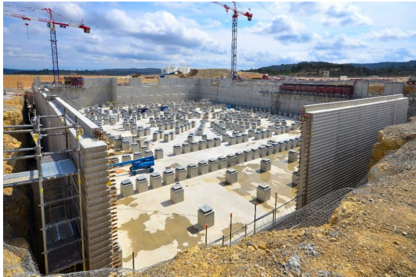
Fig. 8.4-17: First phase works nearly completed in the Tokamak Pit.
