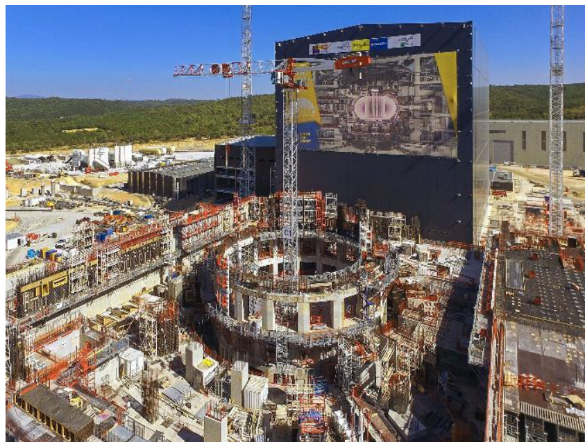
Fig. 8.4-24: The Tokamak Complex "box" as seen by drone.
