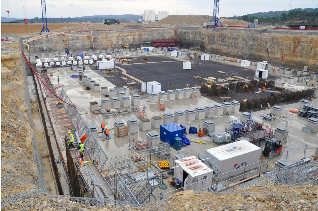
Fig. 8.4-15: Reinforcement work for the basemat of the Tokamak Complex Seismic Pit, November 2011.
