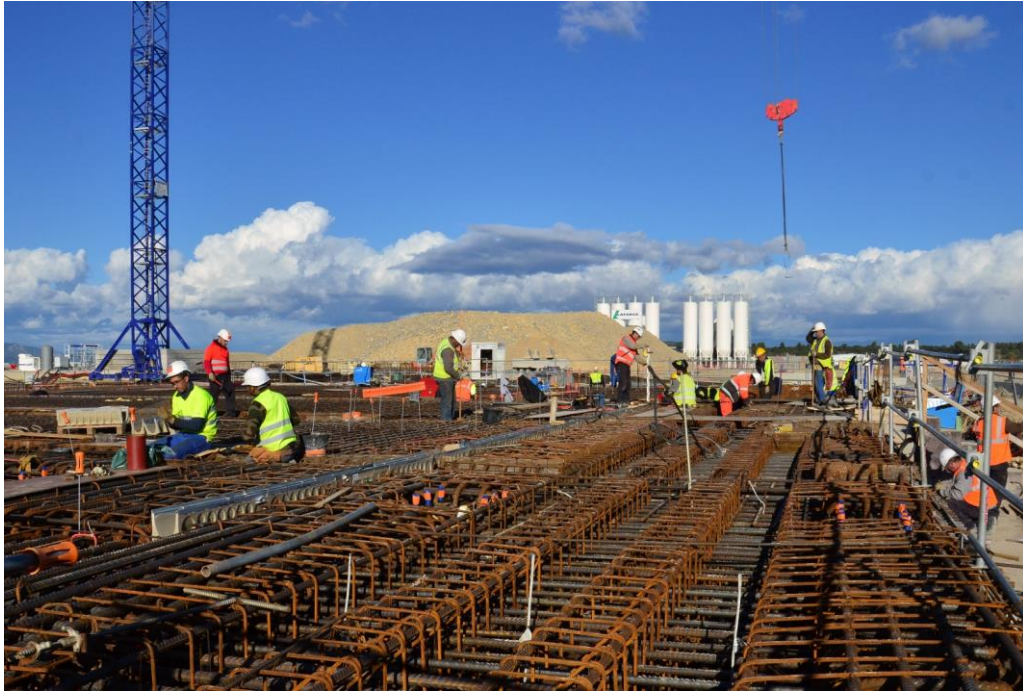
Fig. 8.4-21: Metal "chairs" are positioned on the bottom layer of crisscrossed rebar. Steel reinforcement will be built up to 1.5 metres before foundation pouring begins, June 2012.
