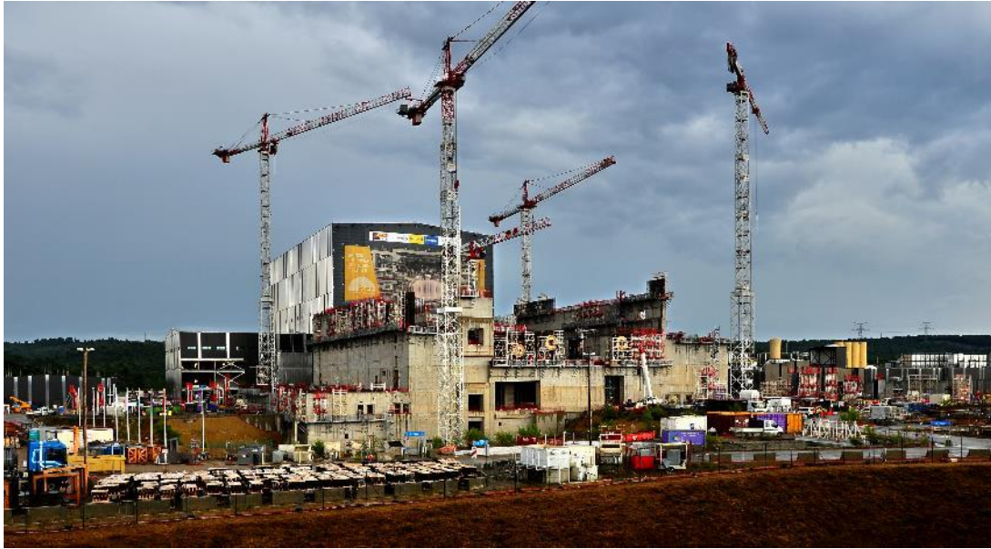
Fig. 8.4-25: Tokamak complex under construction as the clouds roll in, July 2018.
