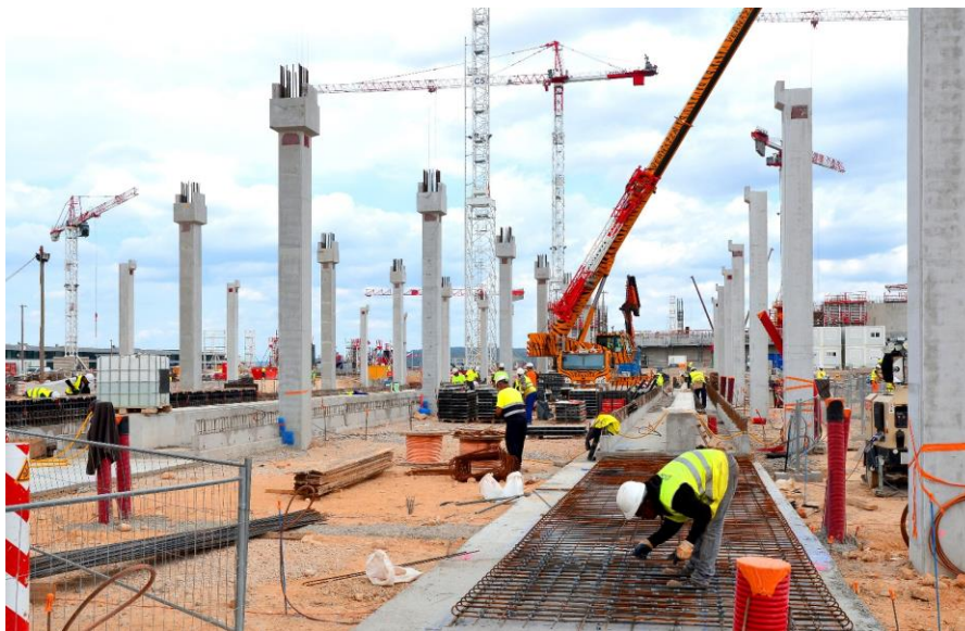
Fig. 8.4-31 : Progress in the conversion building, January 2017.
