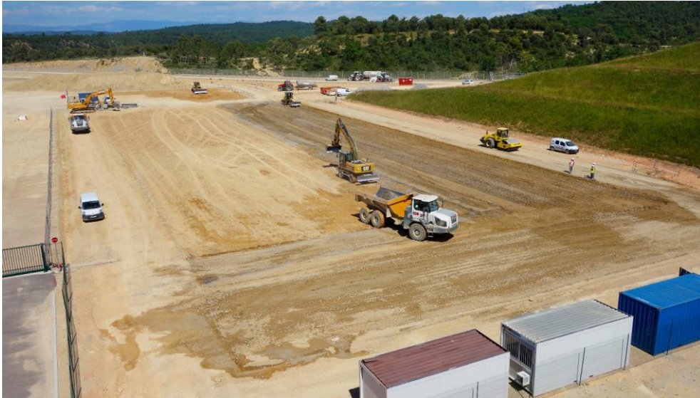
Fig. 8.4-38: The Poloidal Field Winding Facility and the Cryostat Workshop, side by side on the platform, June 2013.
