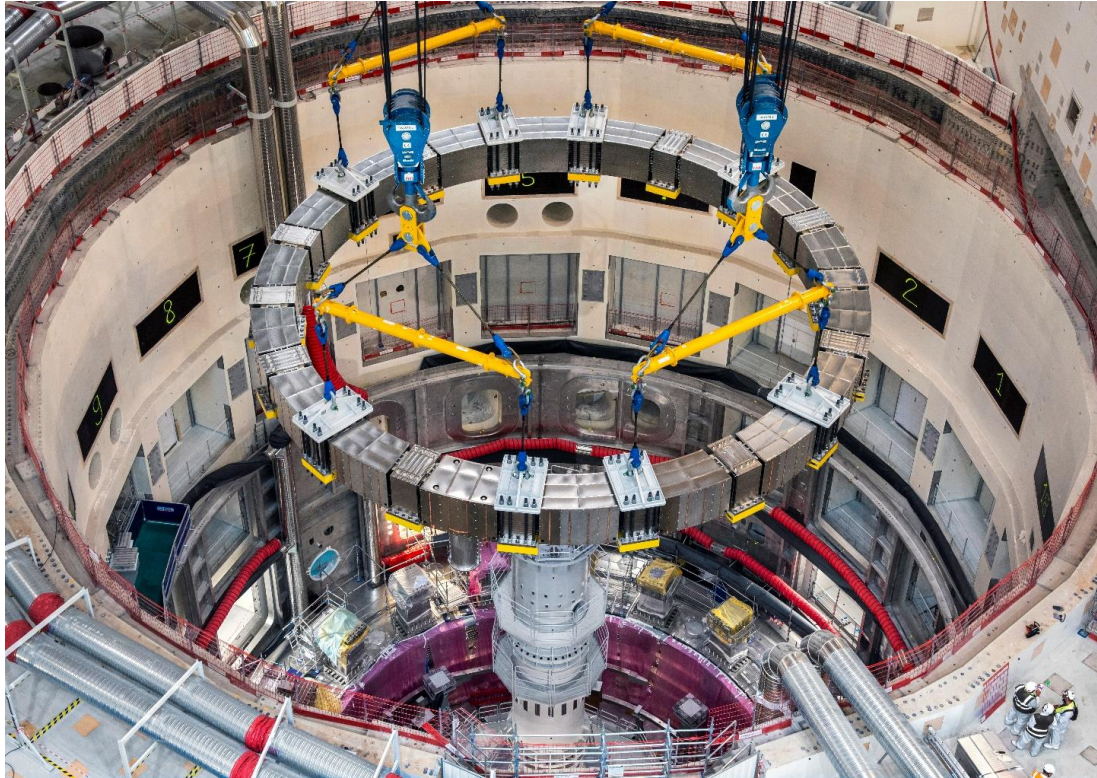
Fig. 8.4-44: The assembly teams lower poloidal field coil #5 into the Tokamak pit.
