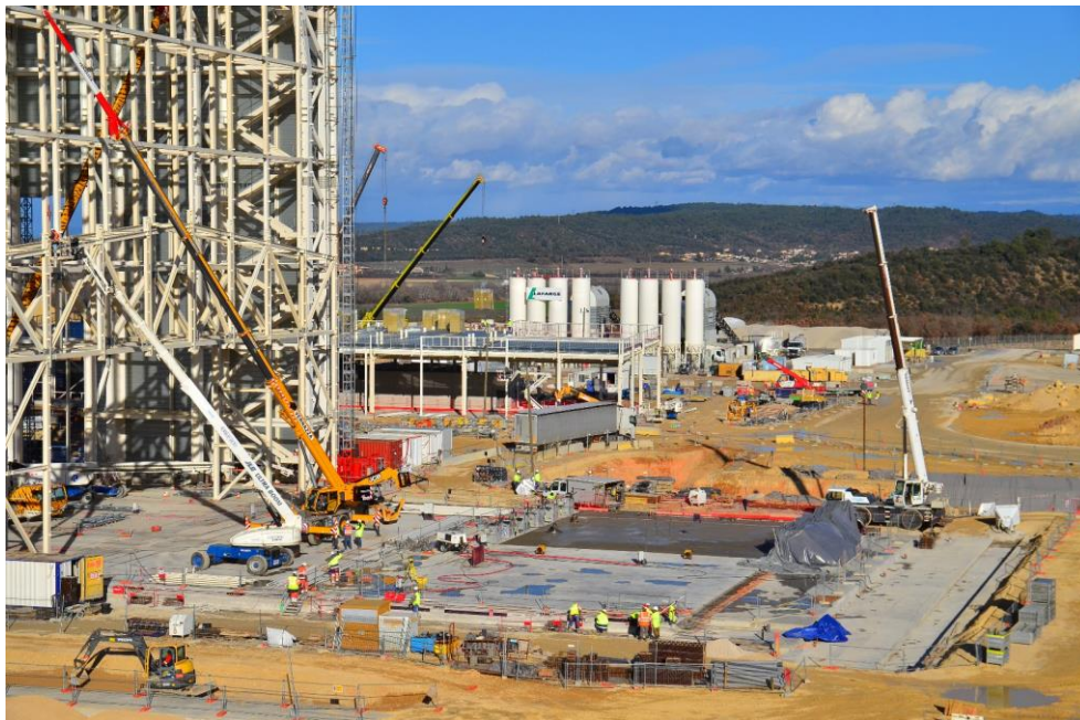
Fig. 8.4-29: Construction of the Cleaning Facility is underway on the south side of the building, Before they enter into the Assembly Hall ITER components will need to be cleaned using a number of different techniques.
