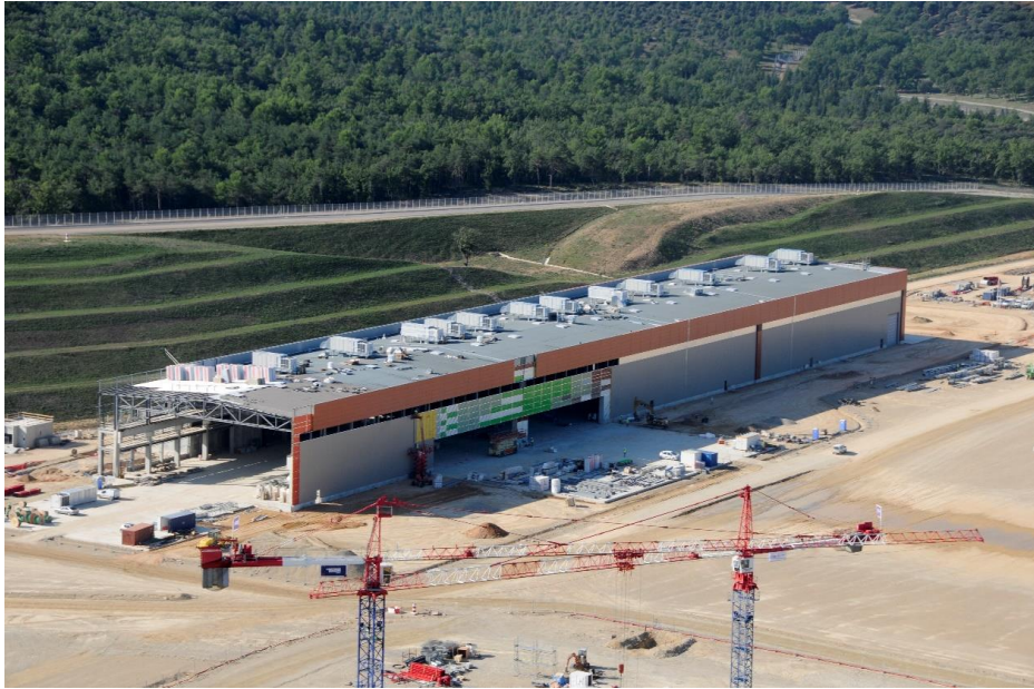
Fig. 8.4-9: The Poloidal Field Coil Winding Facility under construction, exterior work nearly completed.
