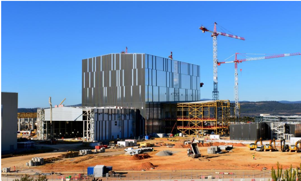
Fig. 8.4-30: The Assembly Hall is joined to two smaller buildings: the Cleaning Facility (left) and the Radio Frequency Heating Building (right).
