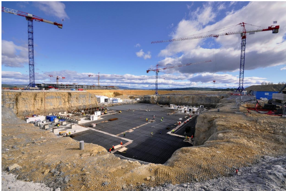
Fig. 8.4-14: Reinforcement work for the basemat of the Tokamak Complex Seismic Pit, October 2011.
