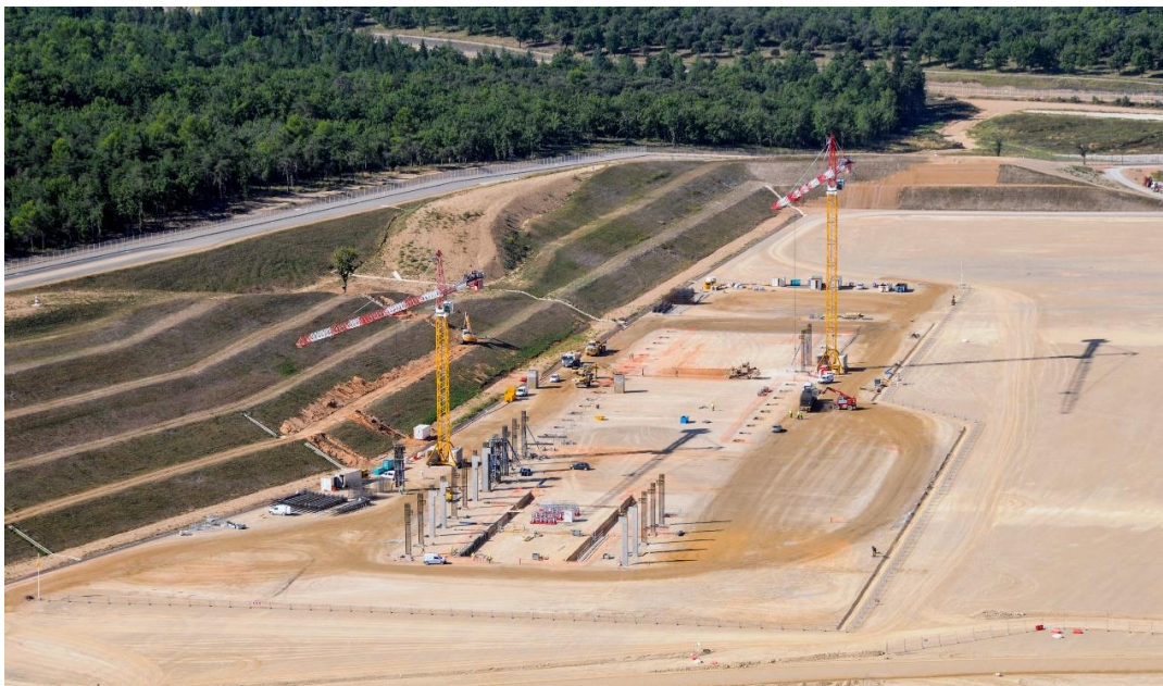
Fig. 8.4-6: The Poloidal Field Coil Winding Facility under construction, lateral view.
