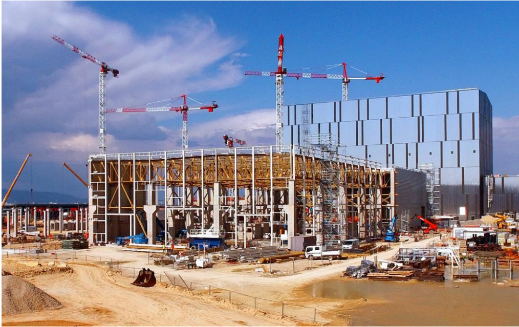
Fig. 8.4-36: Construction of the world's largest concentrated cryoplant is progressing, April 2017.
