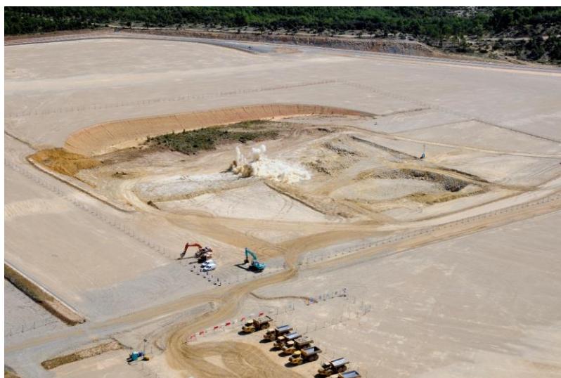
Fig. 8.4-4: Aerial view of the construction site while blasting, September 2010.
