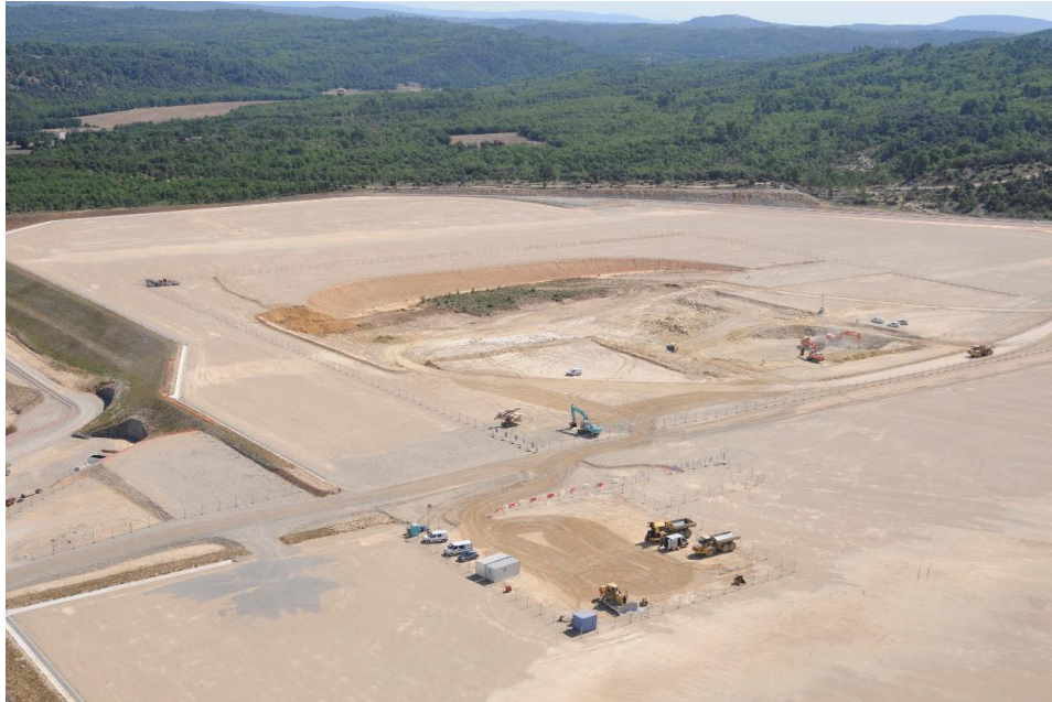
Fig. 8.4-5: Aerial view of the construction site, September 2010.
