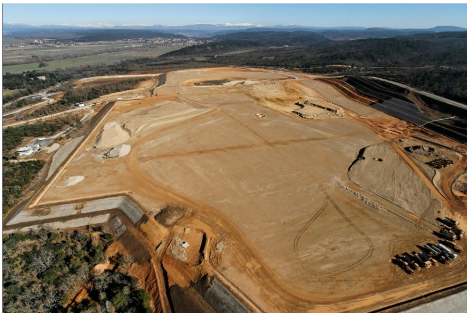
Fig. 8.4-2 : the platform that will house the ITER scientific buildings is ready for construction to begin. 1,000 metres long, 400 me wide.
