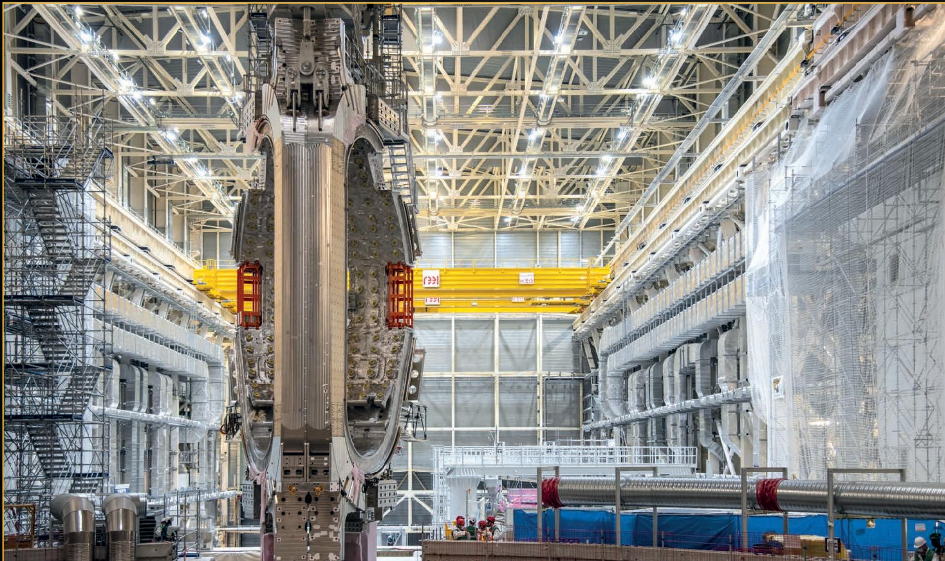
One-ninth of the ITER plasma chamber—a sector module weighing 1,380 tonnes including rigging—is successfully lifted out of tooling and installed in the Tokamak pit on 11 May 2022. The operation, which was months in the planning, went off without a hitch. Eight other similar assemblies will form the complete chamber and surrounding toroidal field coil superstructure. **May 2022**
