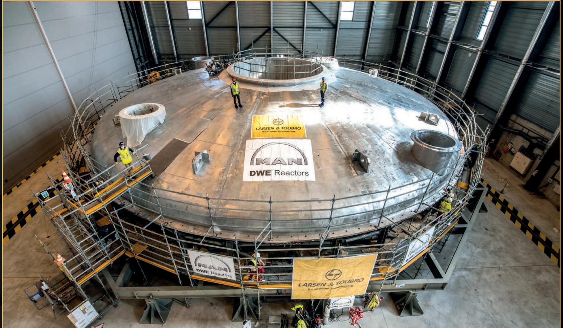
The four sections of the cryostat—the base, lower cylinder, upper cylinder and top lid—have been successively assembled and welded in the on-site Cryostat Workshop from 54 independent segments, each weighing an average of 50 tonnes. With the completion of the top lid (photo), the ITER community celebrates the completion of a yearslong industrial adventure.
