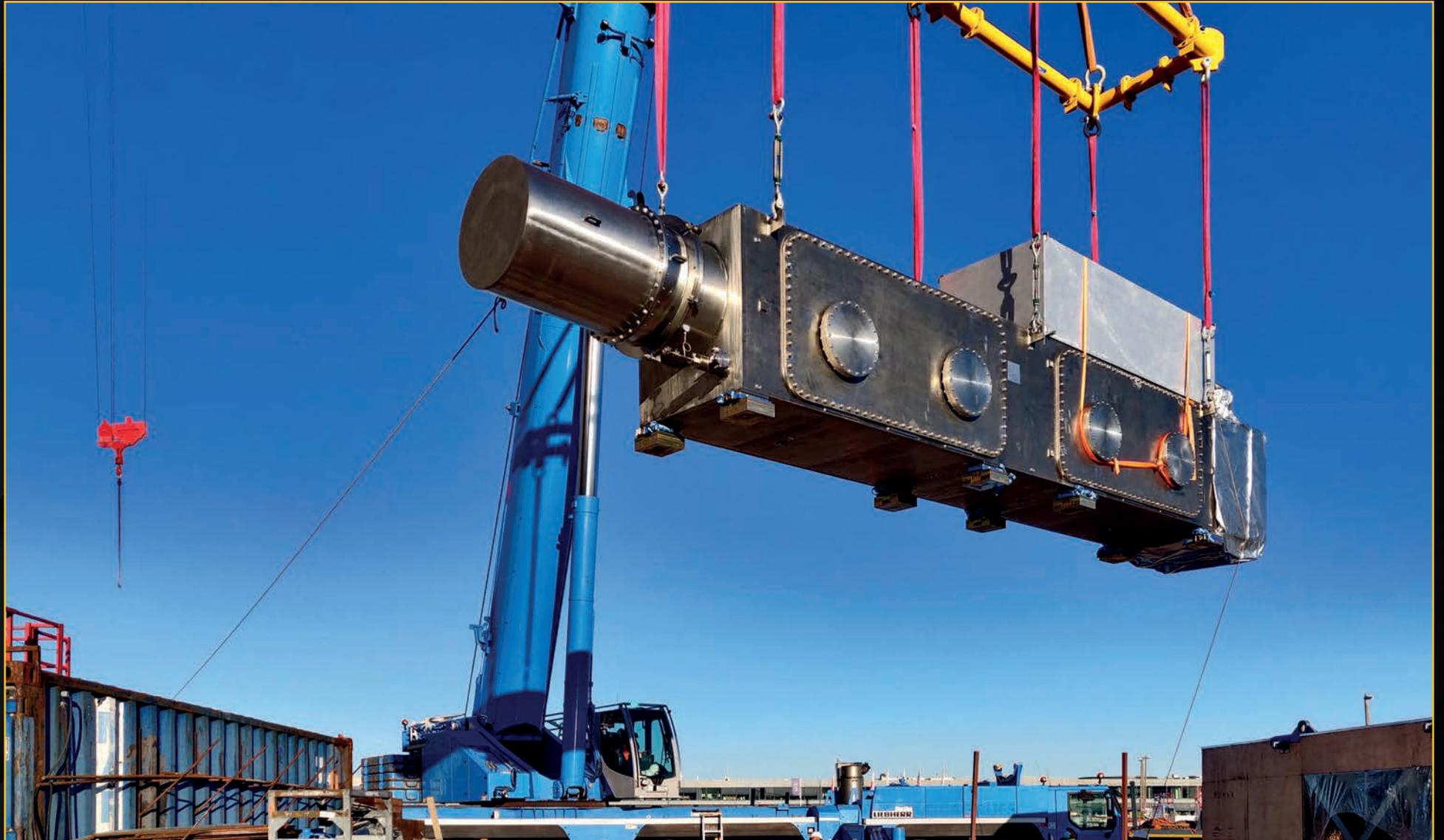
Each of ITER's 31 magnet feeders is produced and shipped in three segments by China. That's approximately 100 feeder large components that must be installed in the Tokamak Complex. **January 2021**
