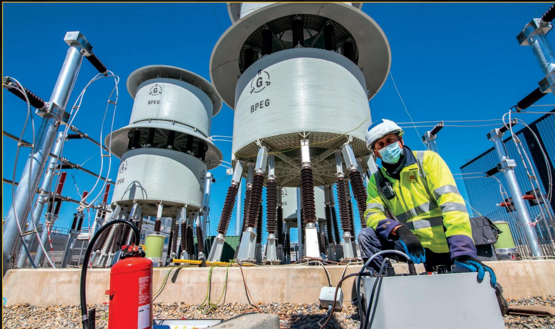
As contractors complete the installation of reactive power compensation and harmonic filtering equipment from China, the focus turns to testing. These 8-metre-tall thyristor-controlled reactors are the first to be energized and put through their paces. **April 2021**
