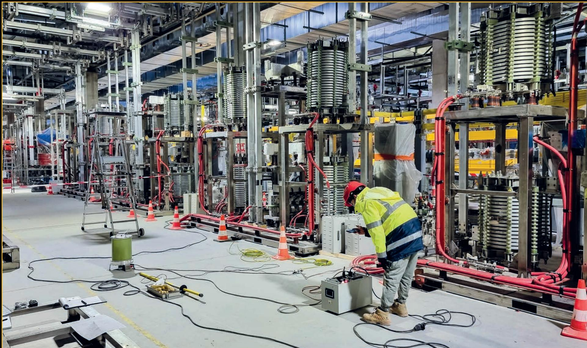
The installation of Korean-made AC/DC converters (17 units) in the Magnet Power Conversion buildings is progressing. This photo shows the insulation voltage test of the AC/DC converters that will provide current to the correction coils.
