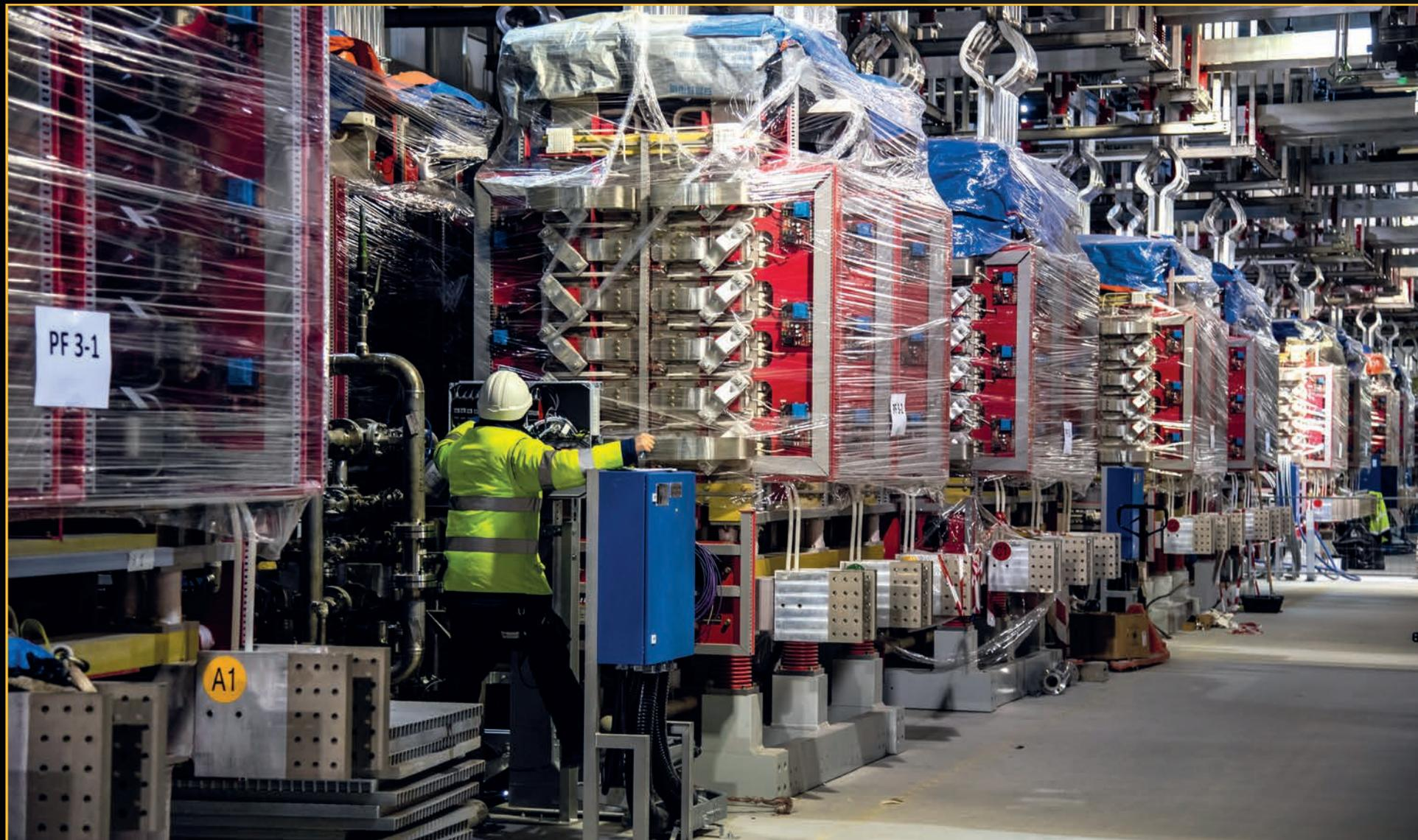
Equipment from China has been installed in the Magnet Power Conversion buildings, which are the «stepping stones» between the power arriving at the ITER switchyard at 400 kV and the voltages required by the ITER magnets. In particular, China has supplied the 14 AC/DC converters that will provide controllable current/voltage to ITER's six poloidal field coils.
