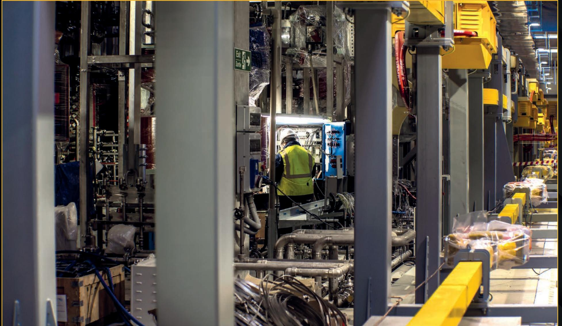
In the ITER Magnet Power Conversion buildings, AC power will be converted into DC current, filtered, and smoothed for the machine's magnetic system. With all equipment installed in one building and 80% in the other, pre-commissioning testing has started. **January 2022**
