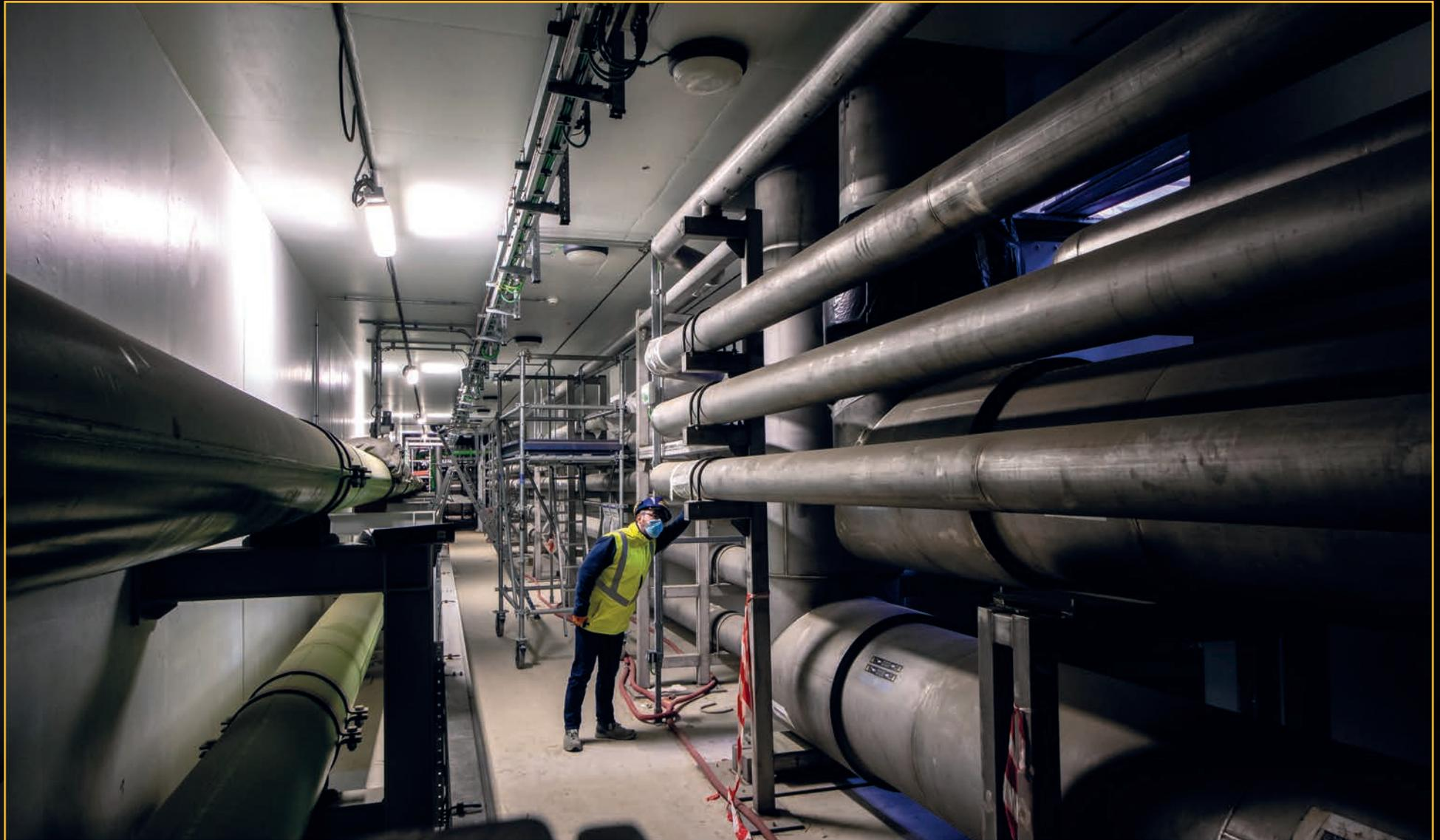
Nearly 25 tonnes of liquid helium at minus 269 °C will circulate in the ITER installation during operation. Four kilometres of process lines like these will carry cryogenic fluids from the cryoplat to clients in the Tokamak Building and back.
