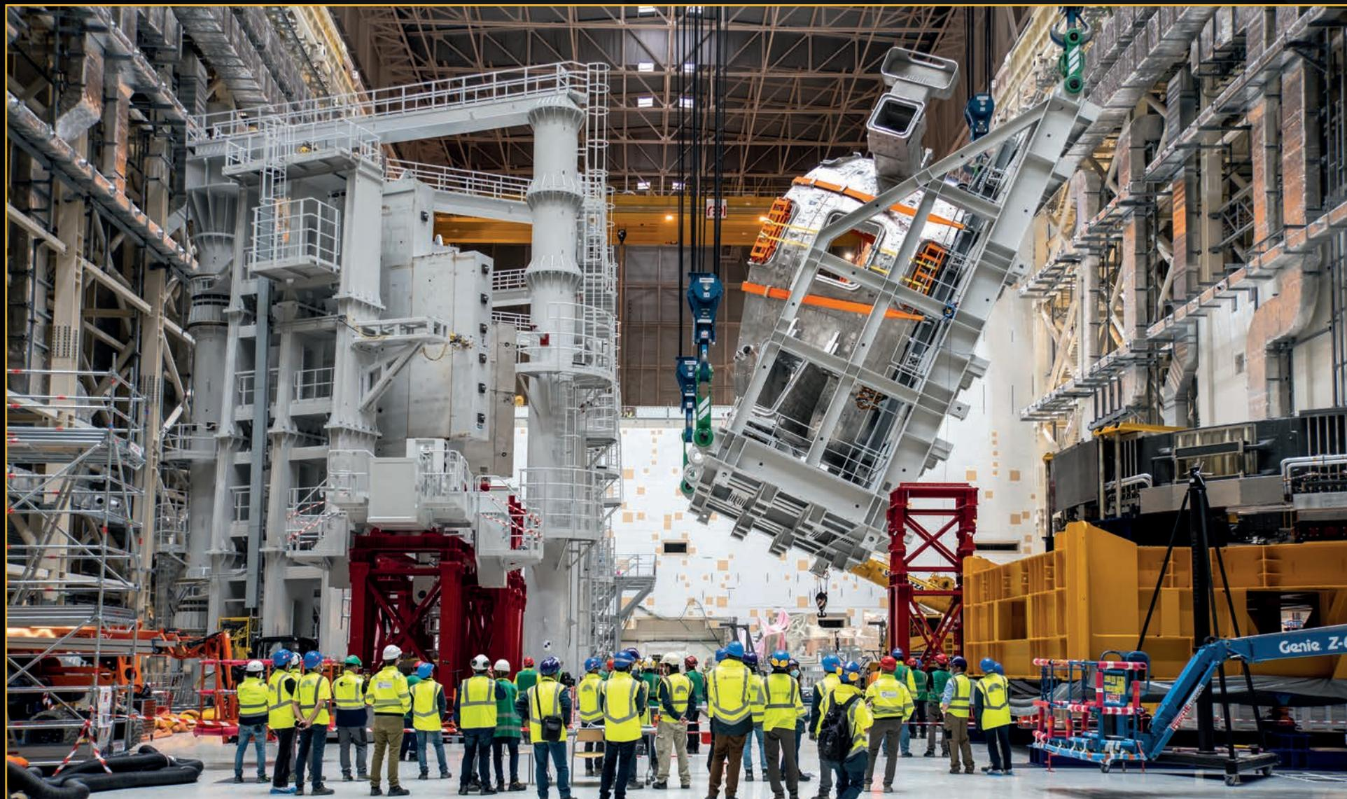
The first vacuum vessel sector to arrive at ITER—sector #6 from Korea—is upended on specialized tooling in March. In this vertical position, it can be installed on sector sub-assembly tooling and prepared for final transfer to the Tokamak pit. **March 2021**
