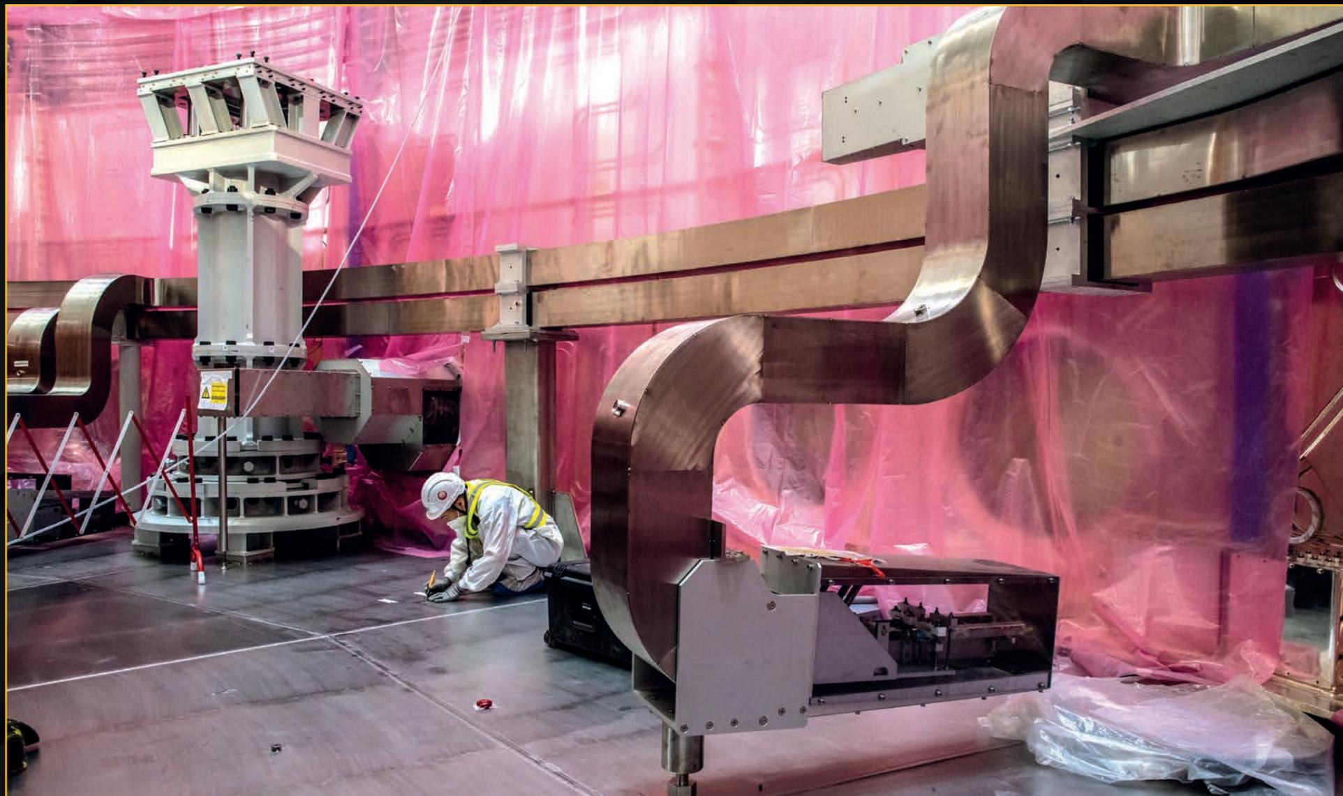
In 2021, the assembly pit is declared "ready" for the first vacuum vessel sector after all captive components (like the magnet feeders pictured here) are installed. **June 2021**
