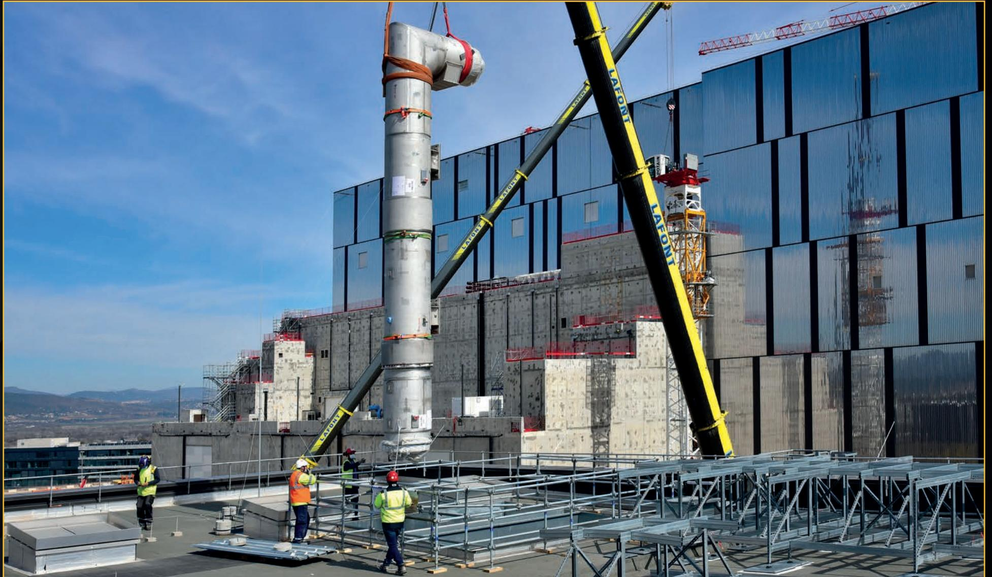
A cryoline spool is installed in the ITER cryoplat, part of the multi-process piping system that will transport cooling fluids to the Tokamak Building. **March 2021**
