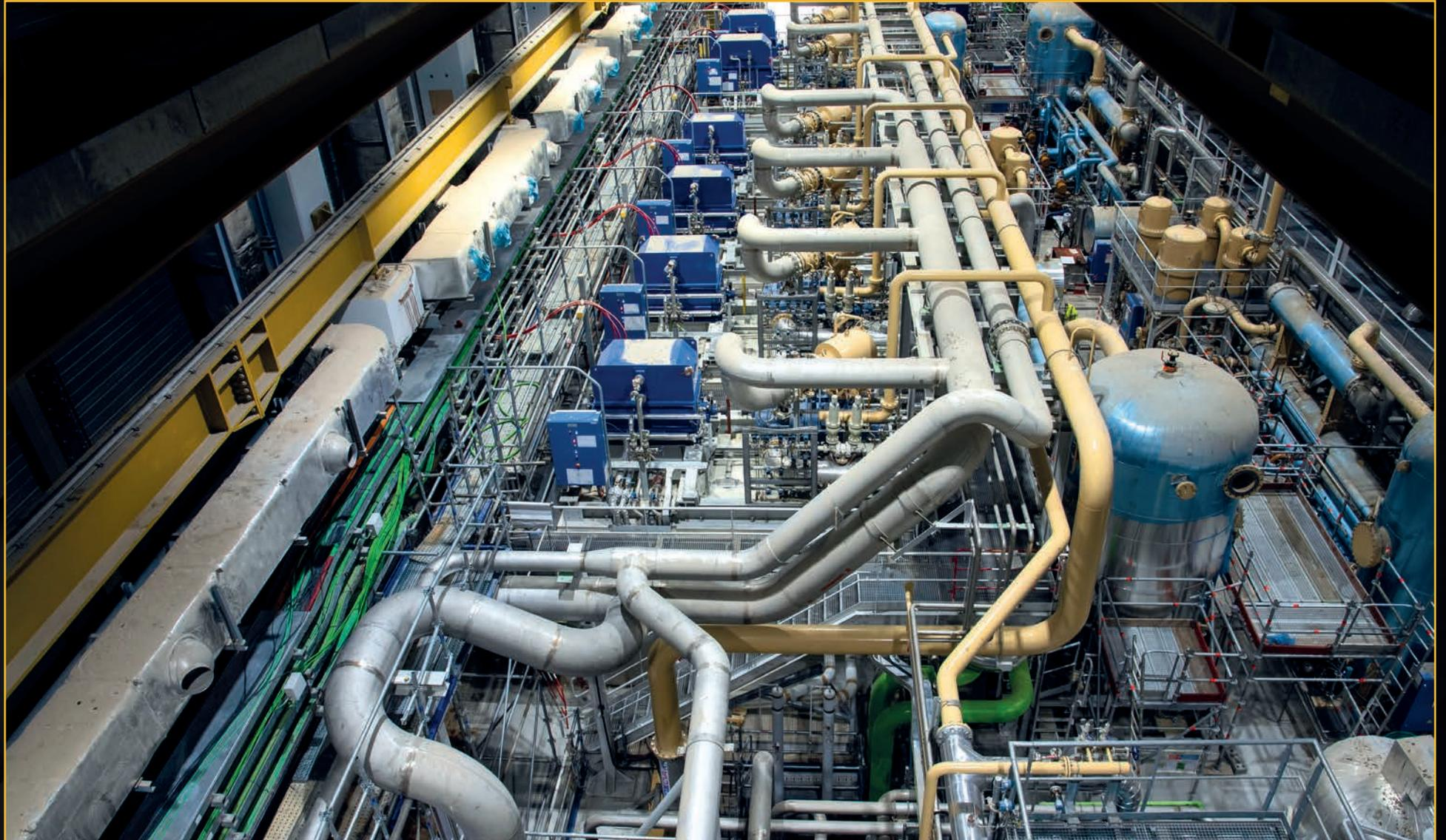
Some 5,000 tonnes of equipment have been installed in the ITER cryoplant. Now, as plant commissioning begins, trucks are rotating on site to fill the exterior tanks with compressed gaseous helium and liquid nitrogen.
