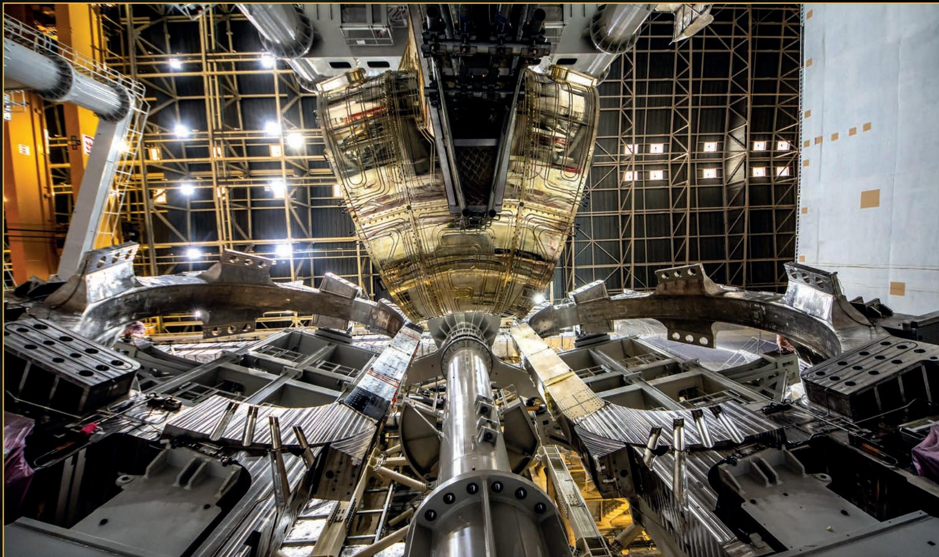
Vacuum vessel sector #6 has been “dressed” in its silver-coated thermal shield but not yet assembled with the two D-shaped vertical coils that are waiting on the wings. Final alignment is achieved in October, as components totalling 1,250 tonnes are aligned to within 1 mm of tolerance in the radial, toroidal and vertical directions. **September 2021**
