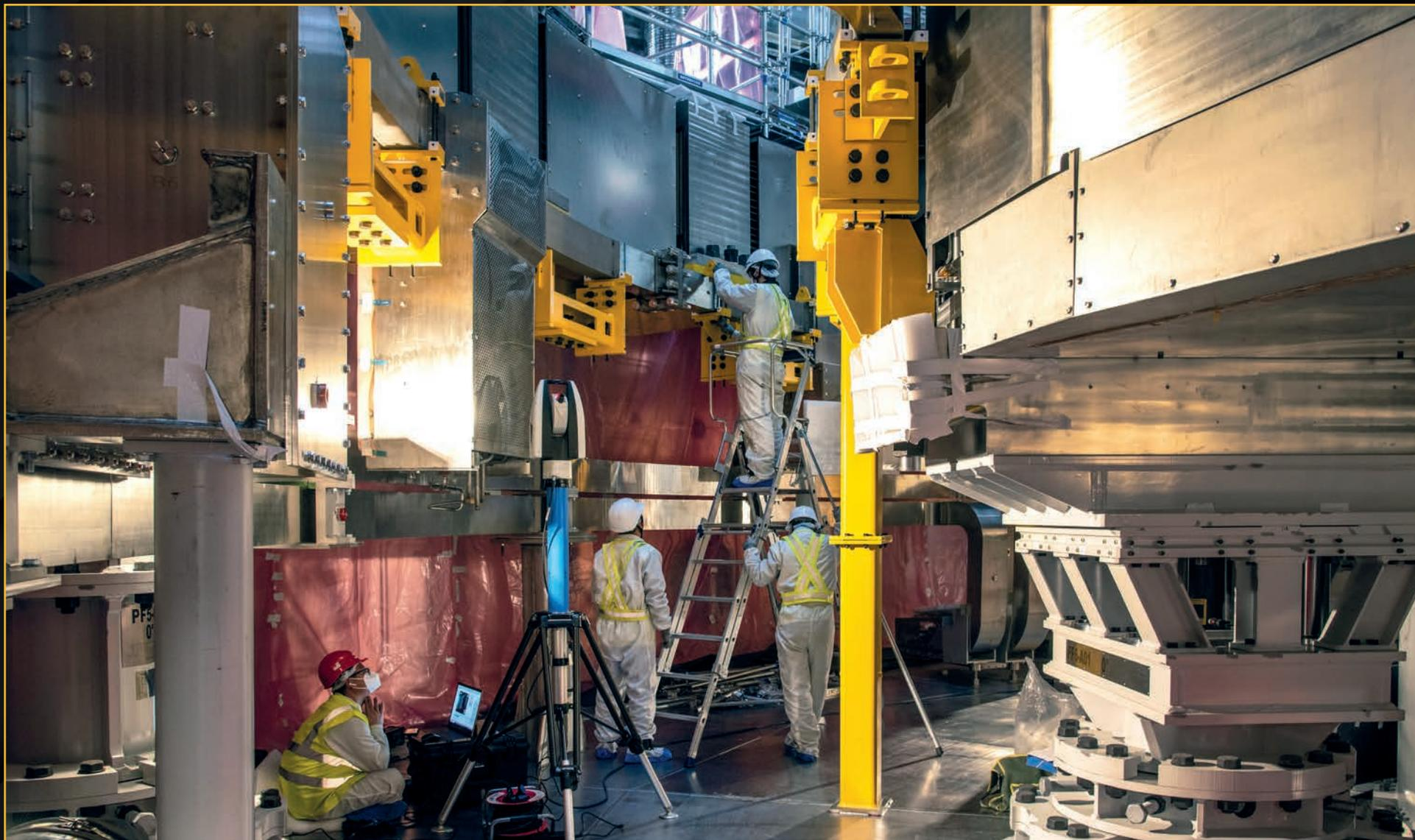
At the very bottom of the Tokamak pit, inside the “soupbowl-like” depression in the cryostat base, teams are installing captive components like the slim magnet feeder lines that will deliver cryogenic fluids and electricity to the lower poloidal field coils. **March 2021**
