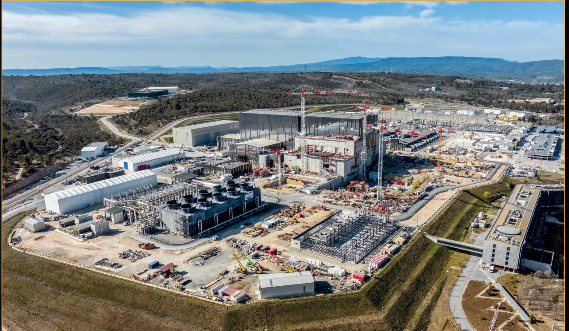
Around the central Tokamak Complex are all of the industrial plant systems—cooling, power, cryogenics, heating, fuel cycle, diagnostics—that enable the operation of the ITER machine. **April 2022**
