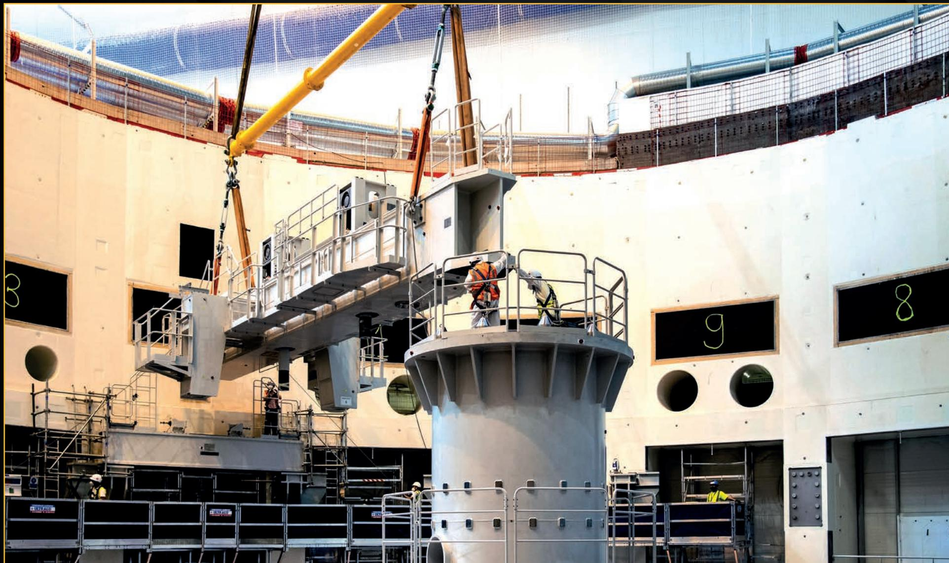
Nine radial beams docked between the central column and brackets on the wall will support the sections of the vacuum vessel as they are welded in the pit. Precise positioning is critical to the alignment of the machine torus. **September 2021**
