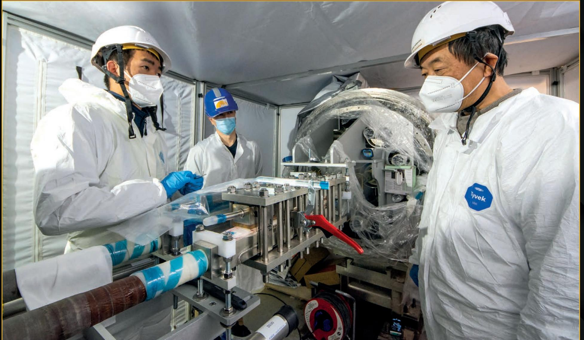
Tokamak assembly is a mix of spectacular operations, such as when giant components are lifted and positioned with complete accuracy, and less visible activities requiring near surgical-like precision. Creating the superconducting joints that join magnet feeder segments (photo) falls into the latter category. **March 2022**
