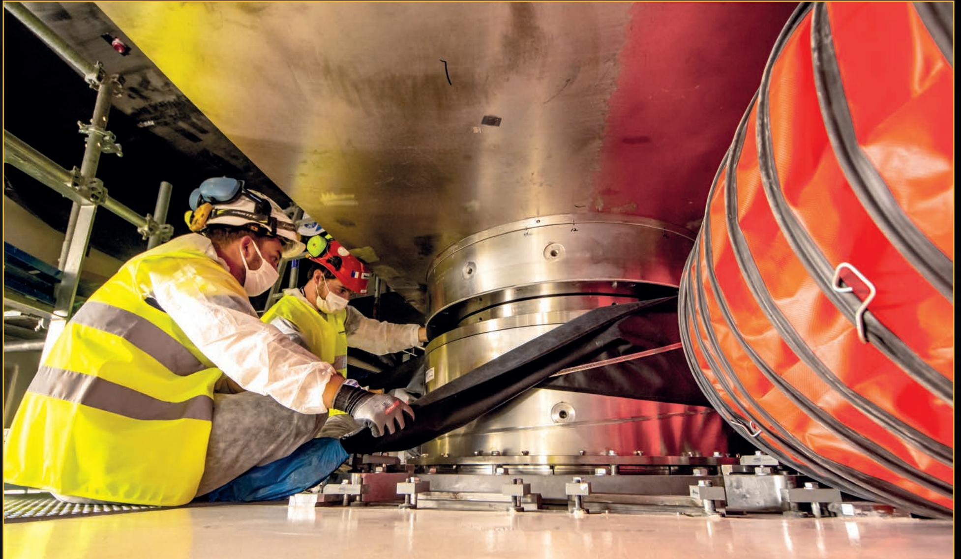
Once installed, components and materials must be kept in good condition until they enter service. Here, a worker performs a white cloth test to check for moisture on a cryostat support bearing during a preservation inspection. **September 2021**
