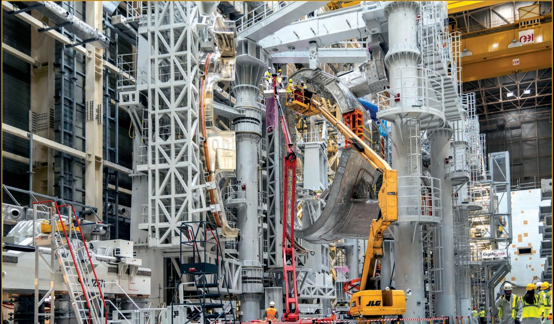
On these twin sector sub-assembly tools in the Assembly Hall, a vacuum vessel sector can be associated with its thermal shield and two toroidal field coils to form a sector module, or one-ninth of the ITER plasma chamber. One sector module was finalized in 2021 and a second is underway. **January 2022**
