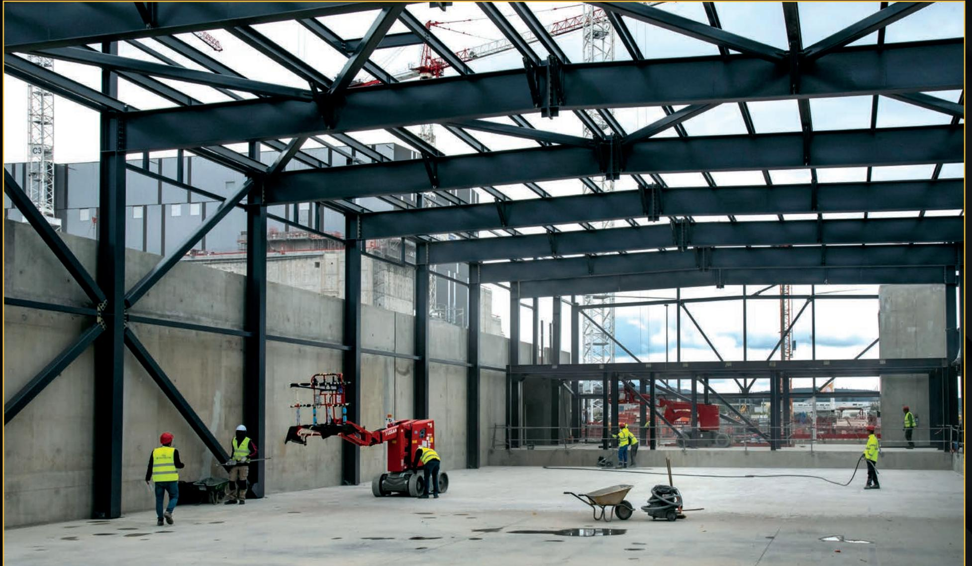
Work is advancing on the ITER Control Building. This 18 m x 43 m space will be the main control room, where scientists, engineers and operators monitor machine operation and analyze the data they receive from each pulse. **May 2022**
