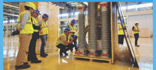
place between the 400 kV switchyard and the transformers that will feed power to the ITER plant systems and components in order to provide protection from the type of major voltage surge that can be caused by lightning.
