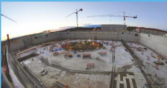
14,000 m<sup>3</sup> of concrete, 3,600 tons of rebar, 8 months of work – the "floor" of the Tokamak Complex was finalized on 27 August 2014.
