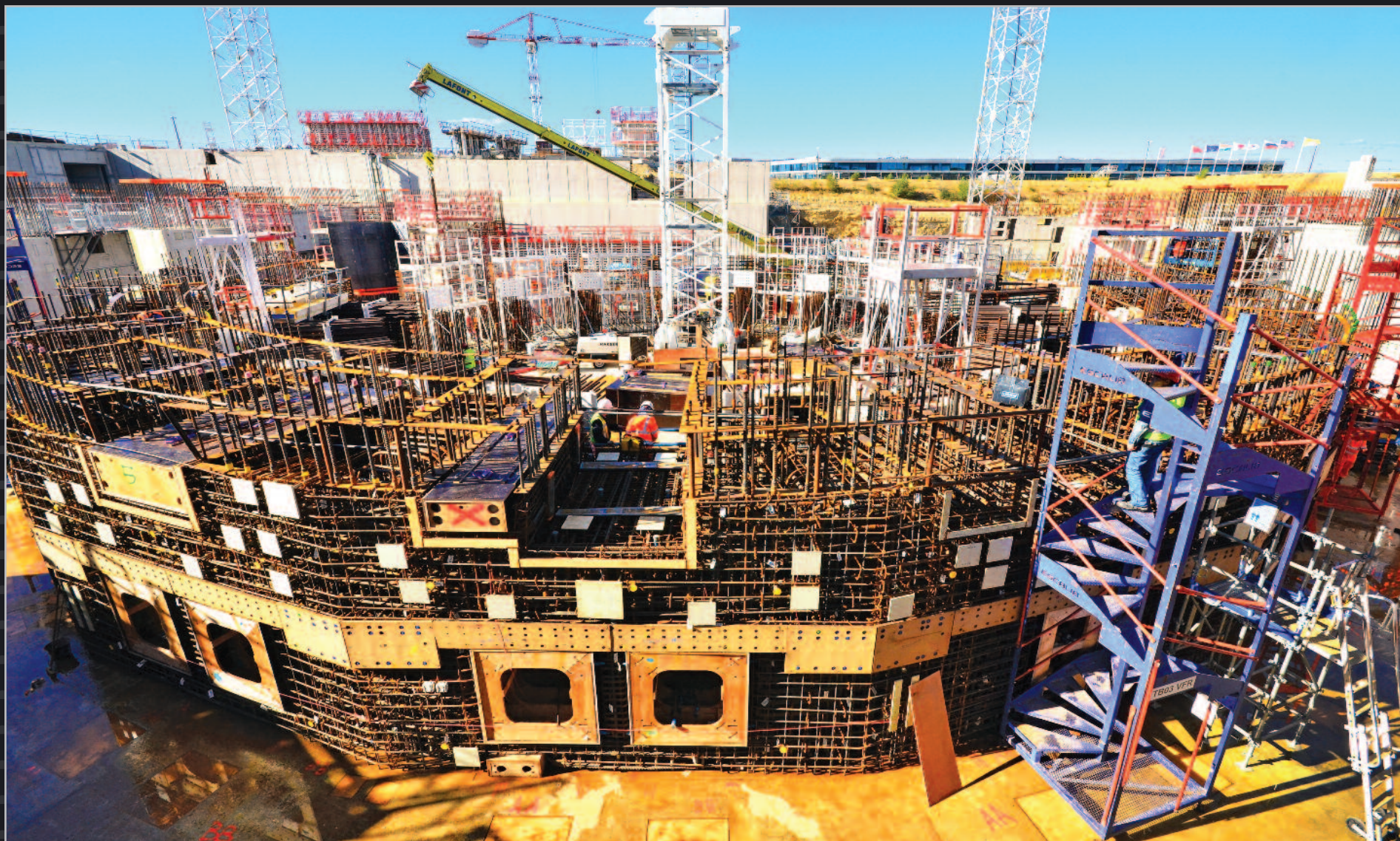
The 3.2-metre-thick ITER bioshield will completely enclose the ITER Tokamak and its cryostat. In the dense reinforcement set into place in advance of concrete pouring, openings are visible for the arrival of electrical and cryogenic supplies. October 2015
