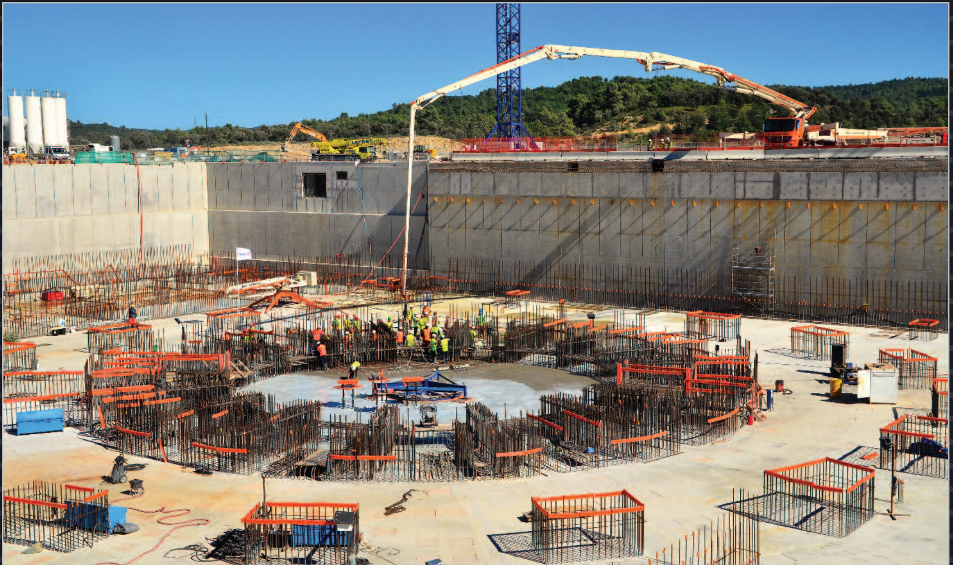
Four years of work in the Tokamak Pit to create the ground support structure and foundations of the Tokamak Complex are brought to a successful conclusion as the last segment of the B2 slab – the basemat that will support the machine and systems – is poured. August 2014
