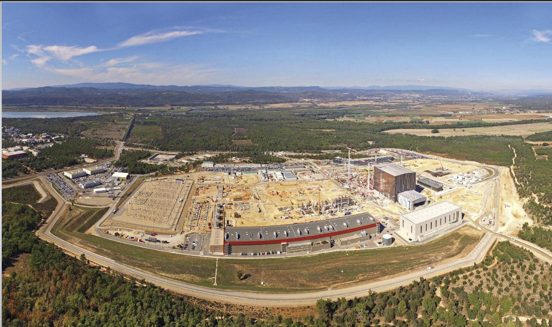
Industrial activity has kicked off in both of ITER's on-site manufacturing facilities: the vast winding facility for poloidal field coils (red trim) where European contractors have installed equipment and begun qualification winding activities; and the Cryostat Workshop (lower right), where Indian contractors have begun welding the cryostat base. October 2016
