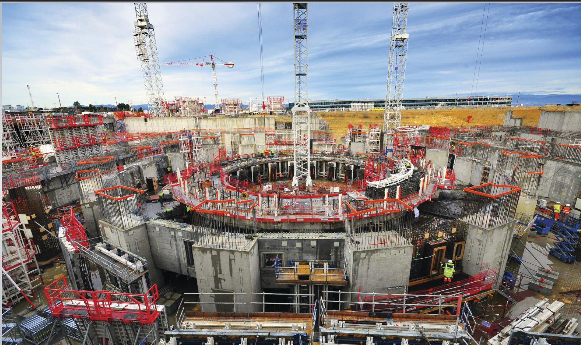
The three-metre-thick ITER bioshield creates an inner circle, with spoke-like reinforcement set in place for the radial walls that will connect it to the cryostat crown. A wider circle is formed by 18 giant columns that will rise 30 metres to provide structural support to the Tokamak Building. January 2016
