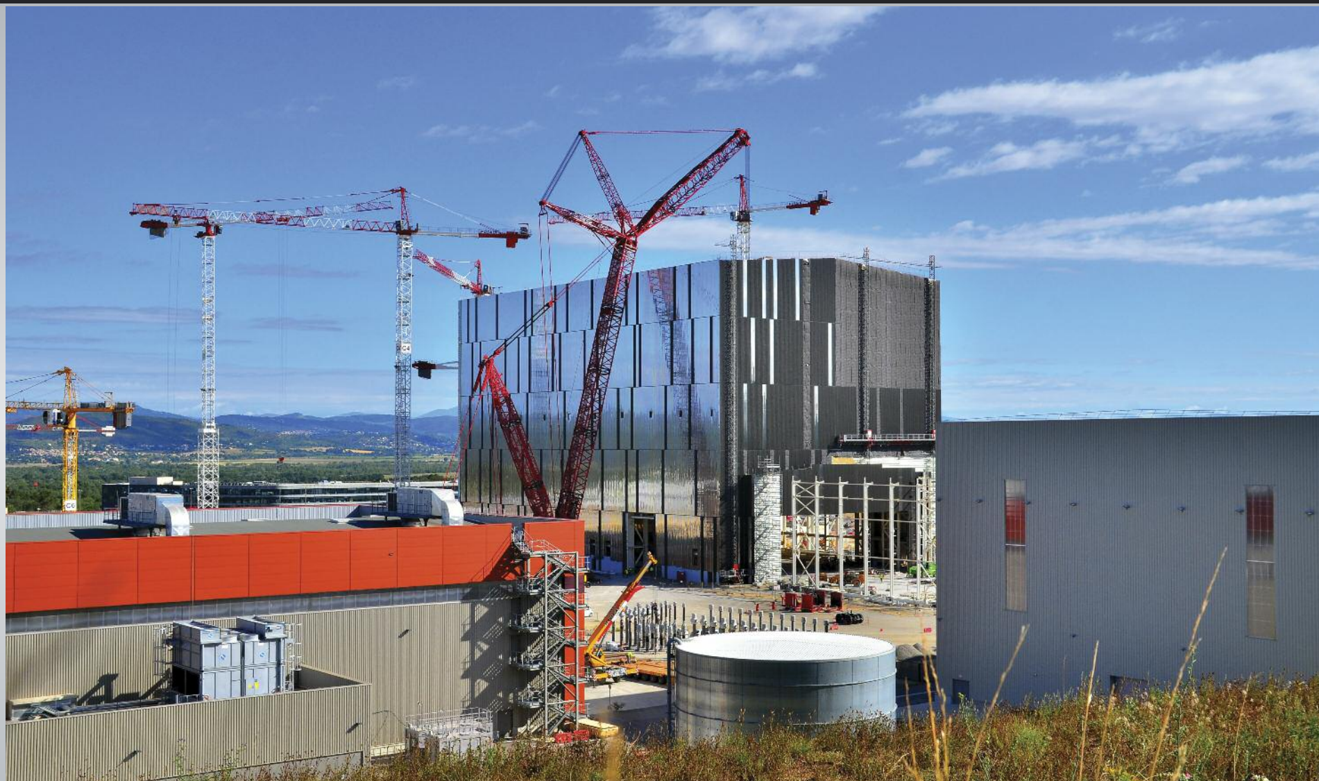
A massive crawler crane raises the four metal girders of the Assembly Hall travelling cranes into position by passing hooks and cables through an opening in the roof. June 2016
