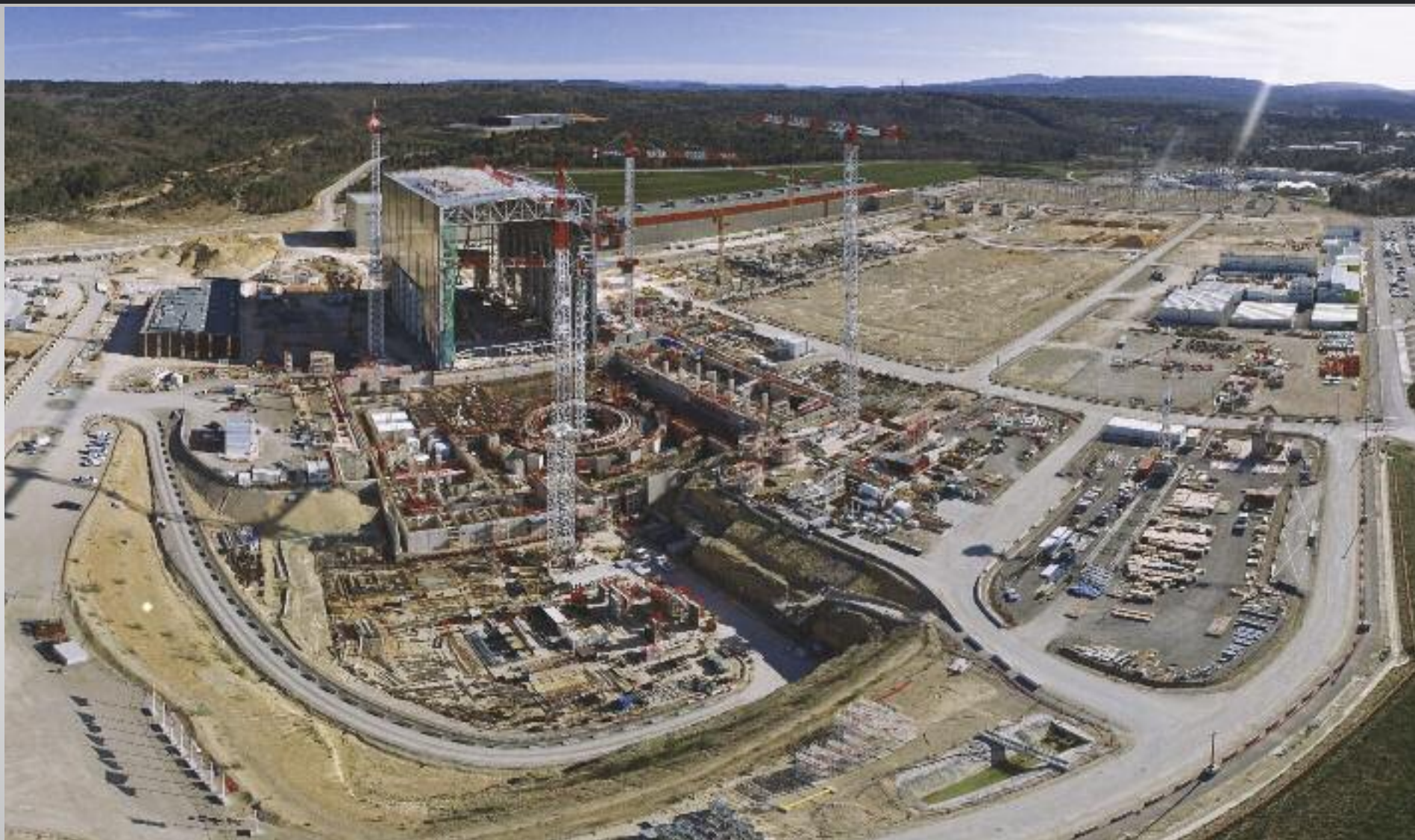
It took four years (2010-2014) to create the foundations of the Tokamak Complex, including the excavation, first-level basemat, retaining walls, seismic pillars and bearings, and second-level basemat. Now, the lowest levels of the Tokamak Complex are taking shape with – at their centre – a perfectly round “well” reserved for machine assembly. April 2016
