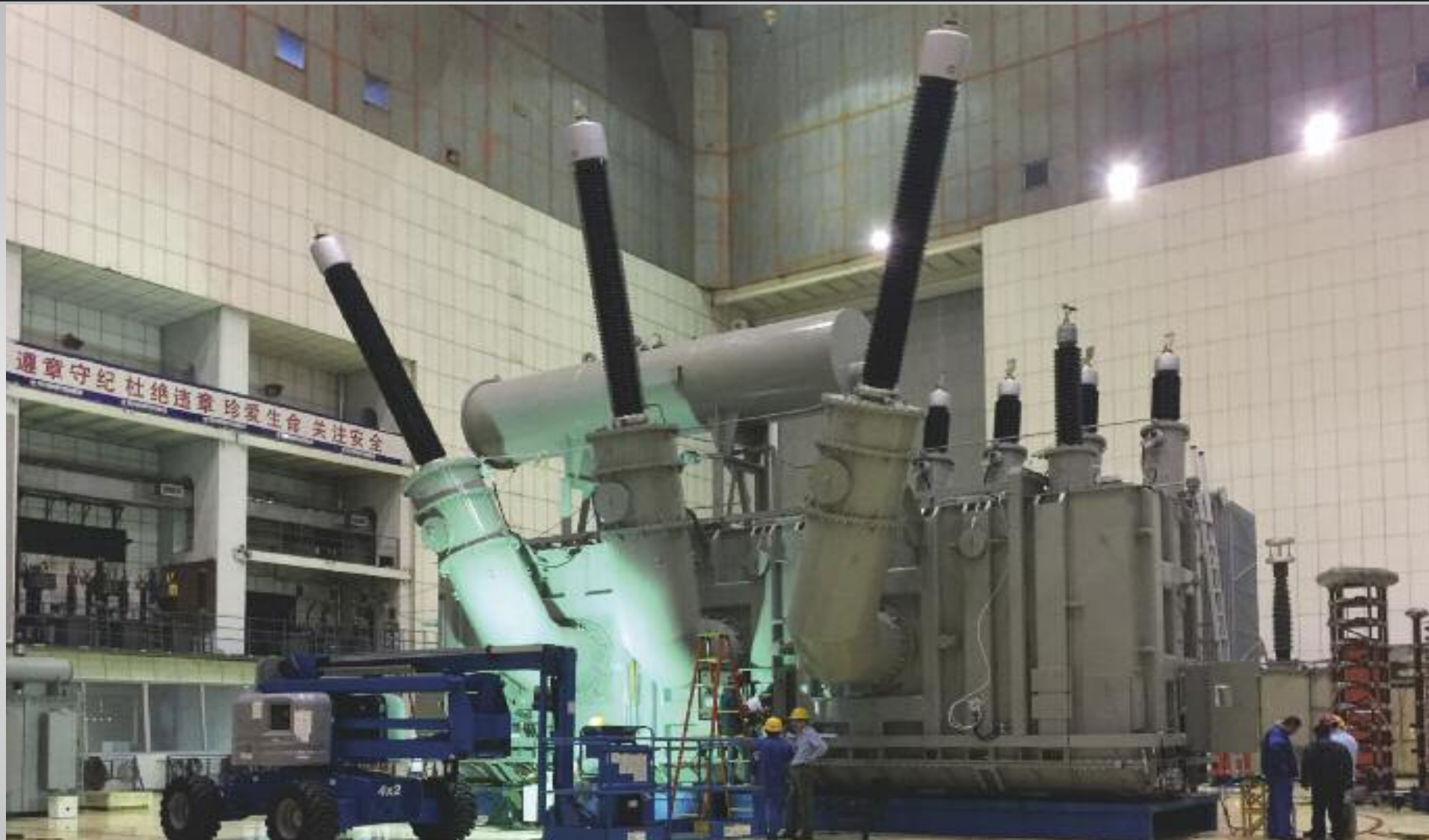
This 300 MVA step-down transformer is one of three that have successfully passed factory acceptance tests in China for ITER's pulsed power electrical network. The first transformer reached ITER in 2016; two others are expected next year.
