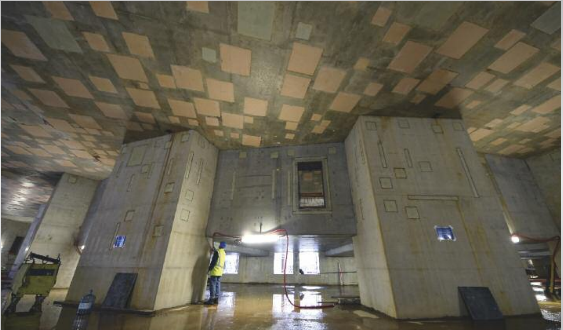
The cavernous area in the basement of the Tokamak Building will completely fill up with pipes, cables, feeders and busbars as the Tokamak systems are installed. The equipment will be anchored to the embedded plates that can be seen in the floor, walls and ceiling. October 2016
