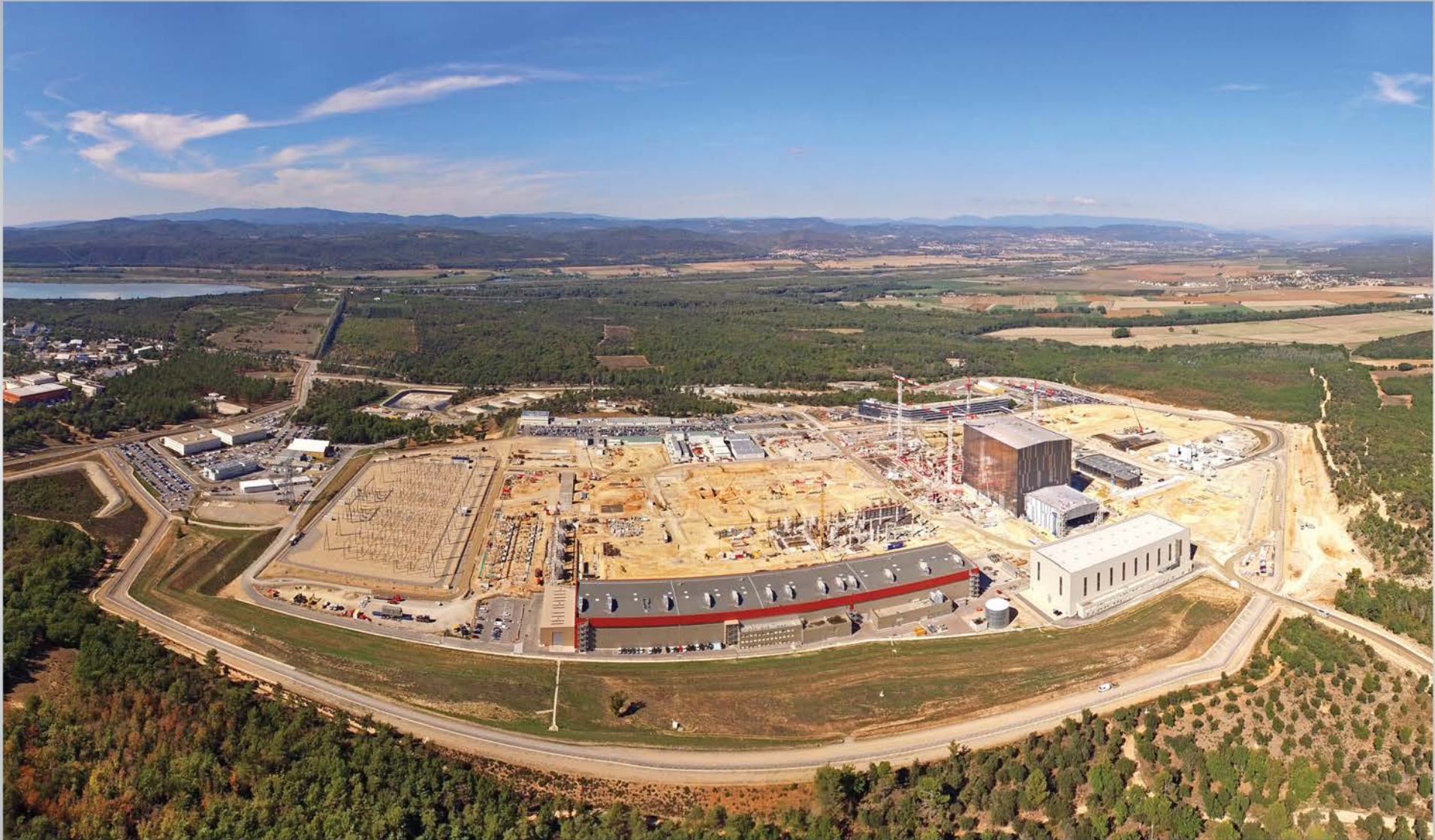
Industrial activity has kicked off in both of ITER's on-site manufacturing facilities: the vast winding facility for poloidal field coils (red trim) where European contractors have installed equipment and begun qualification winding activities; and the Cryostat Workshop (lower right), where Indian contractors have begun welding the cryostat base. October 2016
